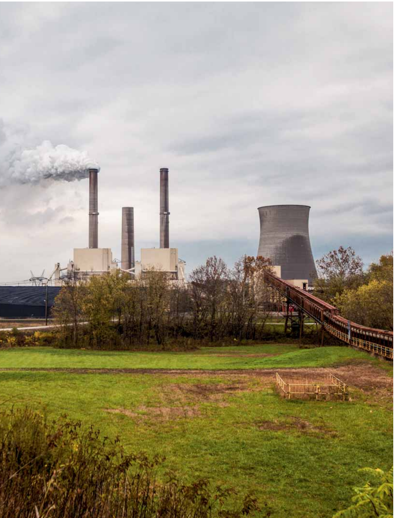
The Gavin Plant was one of several to add flue gas scrubbers in its smokestacks.
