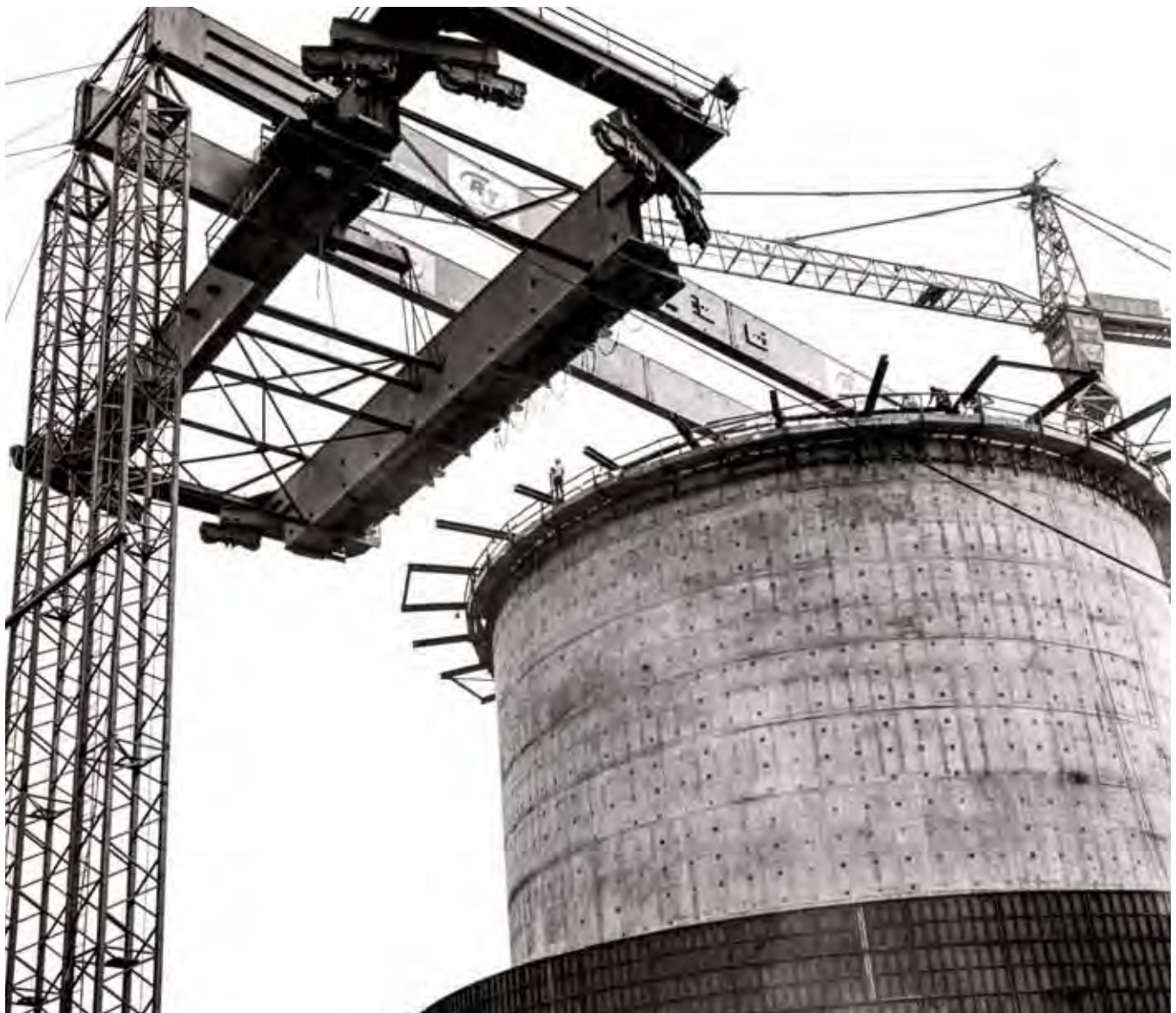
Positioning of nuclear reactor at Cook Plant
