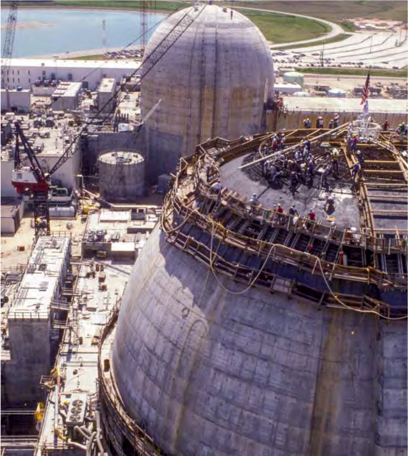
South Texas Dome construction, late 1970s
