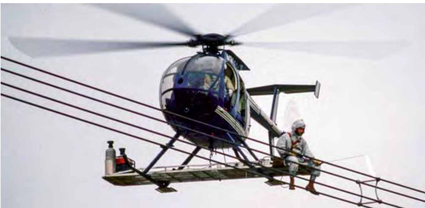
A line mechanic working on a live wire from a helicopter platform
