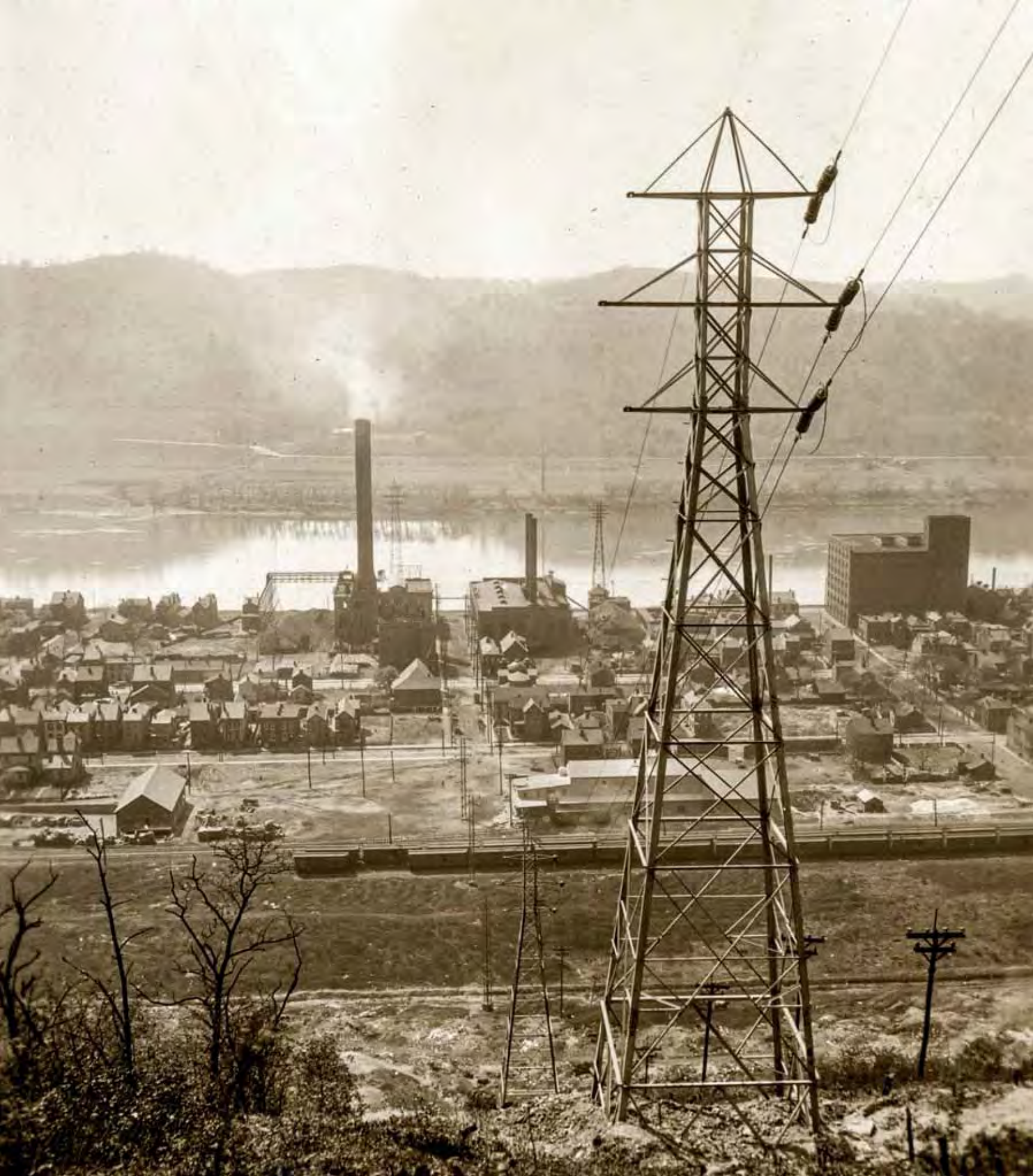
Overlooking the city of Wheeling, West Virginia, with newly erected 138-kilovolt transmission towers for growing demand
