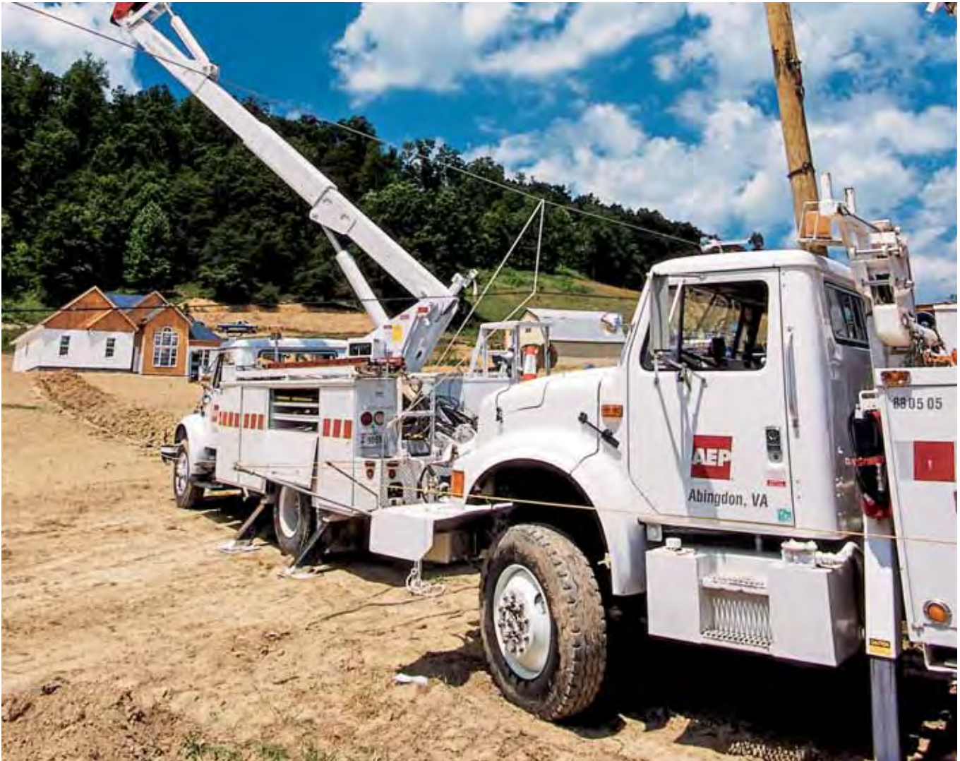
New line installation in Abingdon, Virginia
