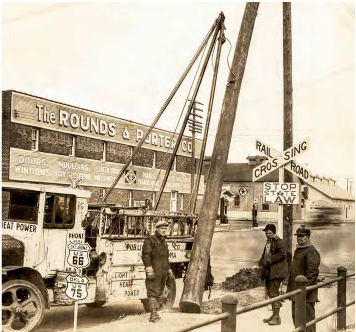
PSO line crew putting up a new pole in Tulsa, c. 1924
