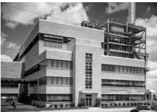
Renovated Corpus Christi Plant
