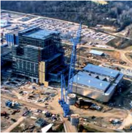
Construction on the conversion of the Zimmer Plant
