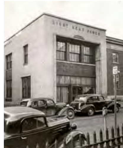
The Welch office, one of several offices of Appalachian Power acquired by AGE
