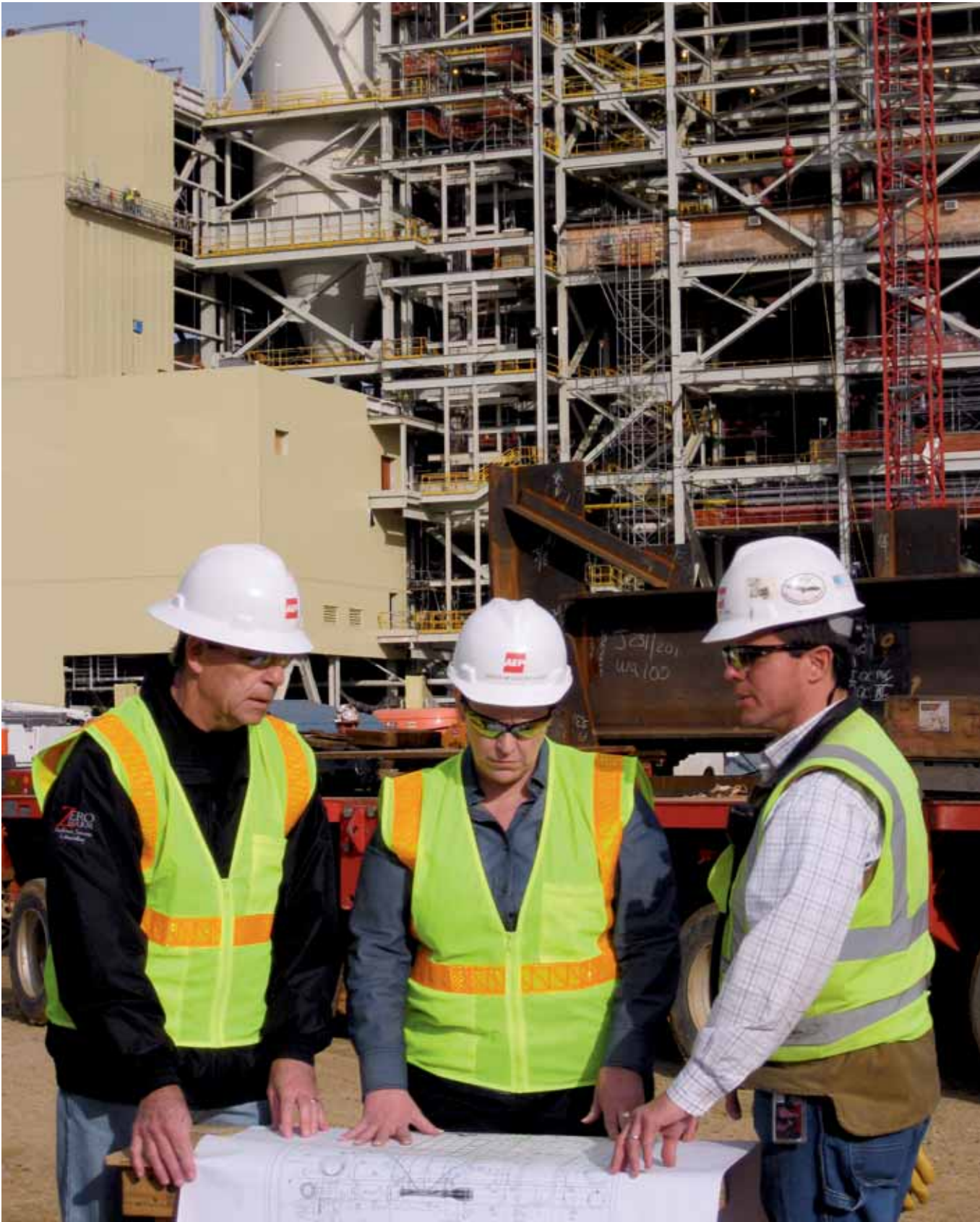
Turk Power Plant construction, Fulton, Arkansas
