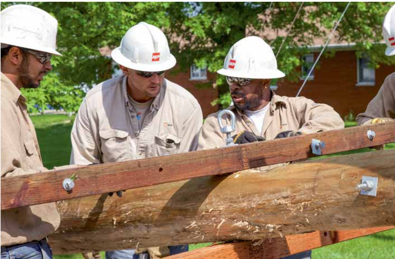
AEP Ohio line mechanics prepare to install a utility pole.
