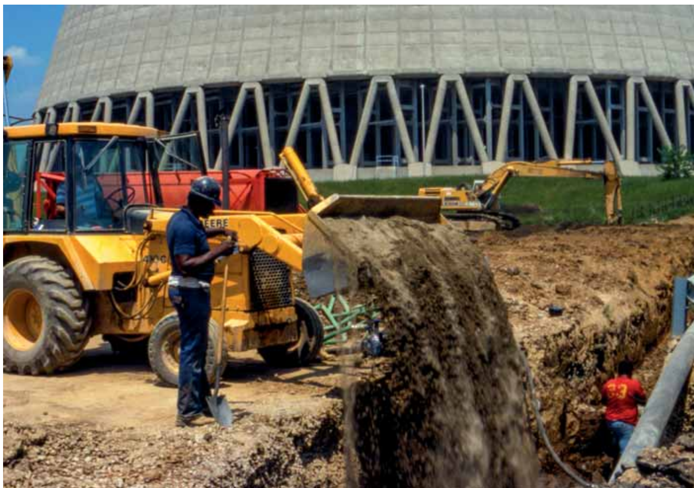
Construction of the William H. Zimmer Plant, Moscow, Ohio
