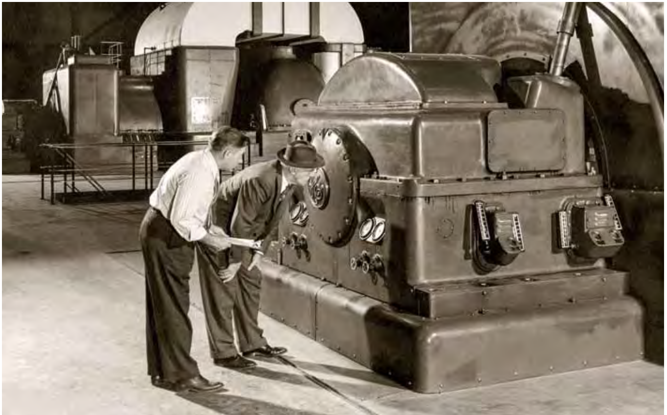
Philip Sporn inspects equipment at the plant named after him.
