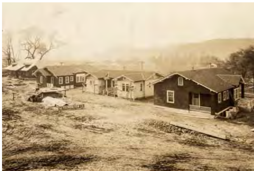
Windsor Plant housing
