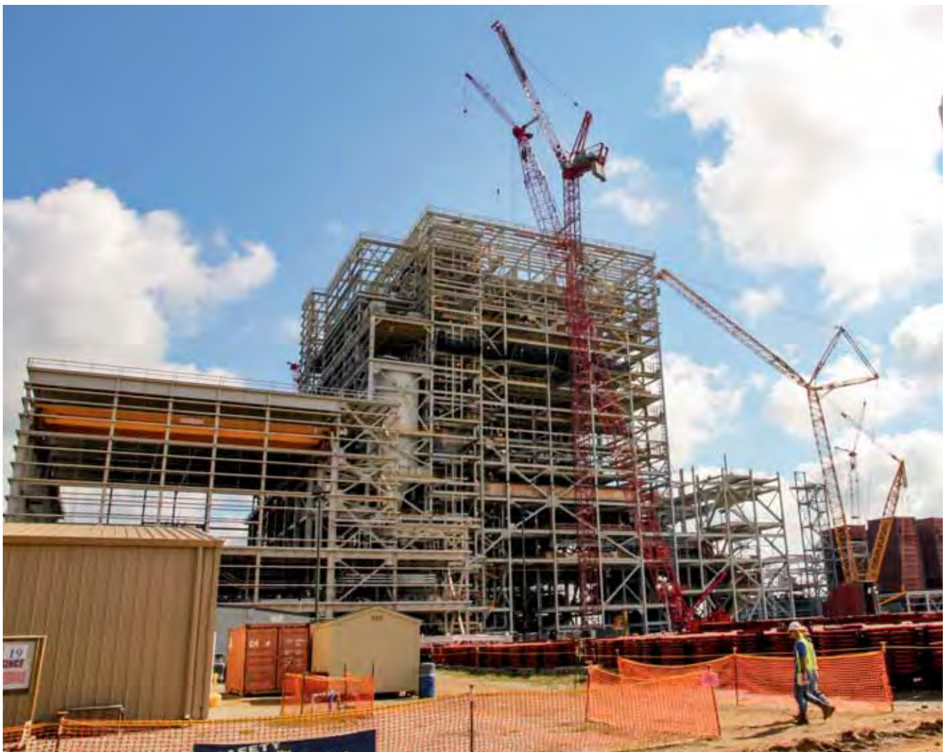
Construction of AEP's award-winning Turk Plant, the industry's first ultra-supercritical plant
