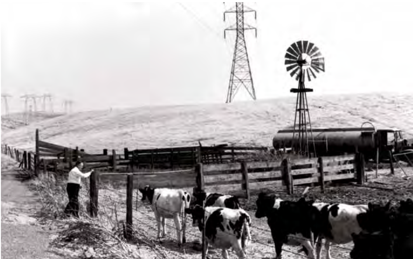
West Texas Utilities' Fort Davis transmission lines at Altamont Pass
