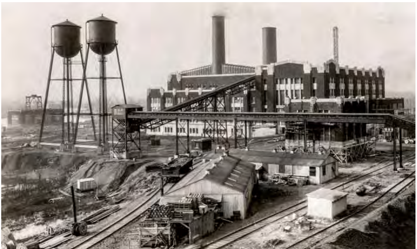
The Twin Branch Plant
