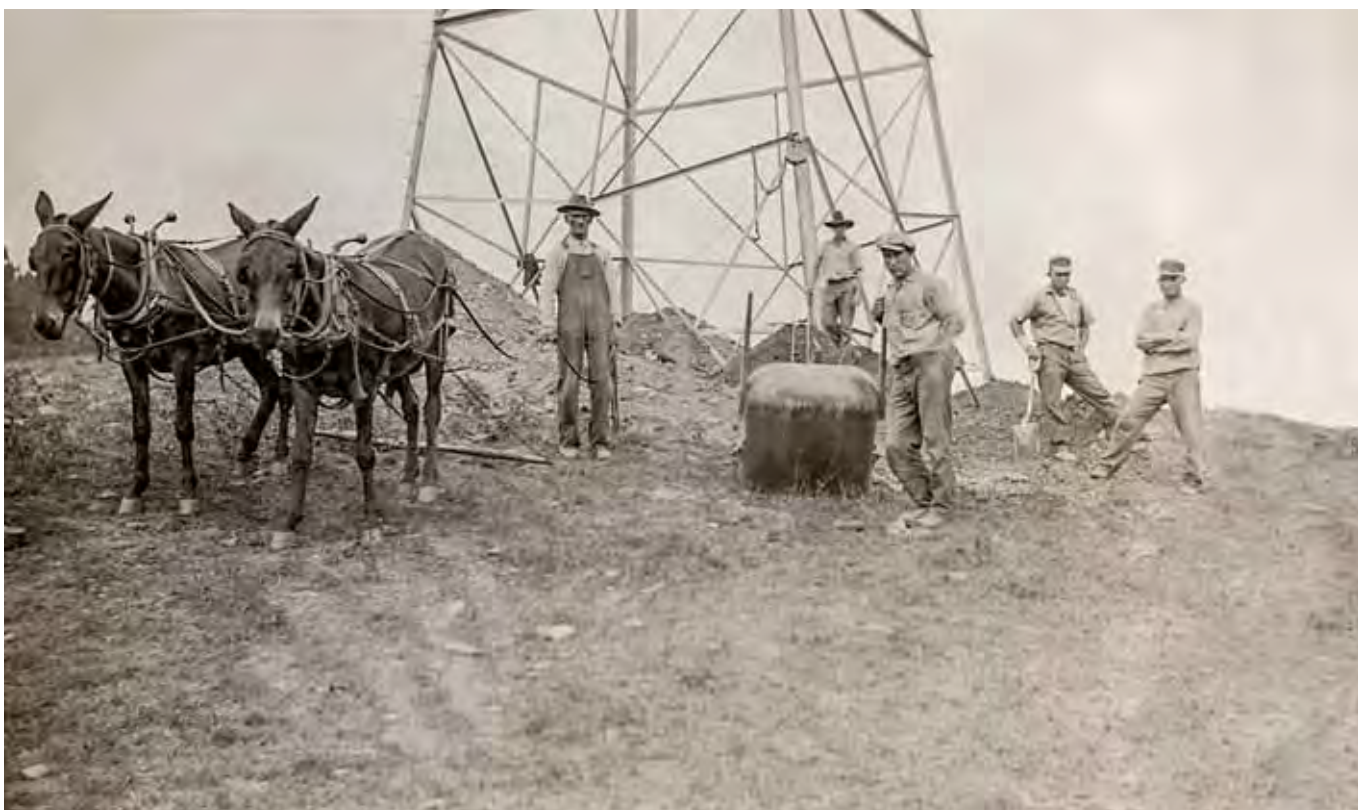
Backfilling crew on tower construction, 1925
