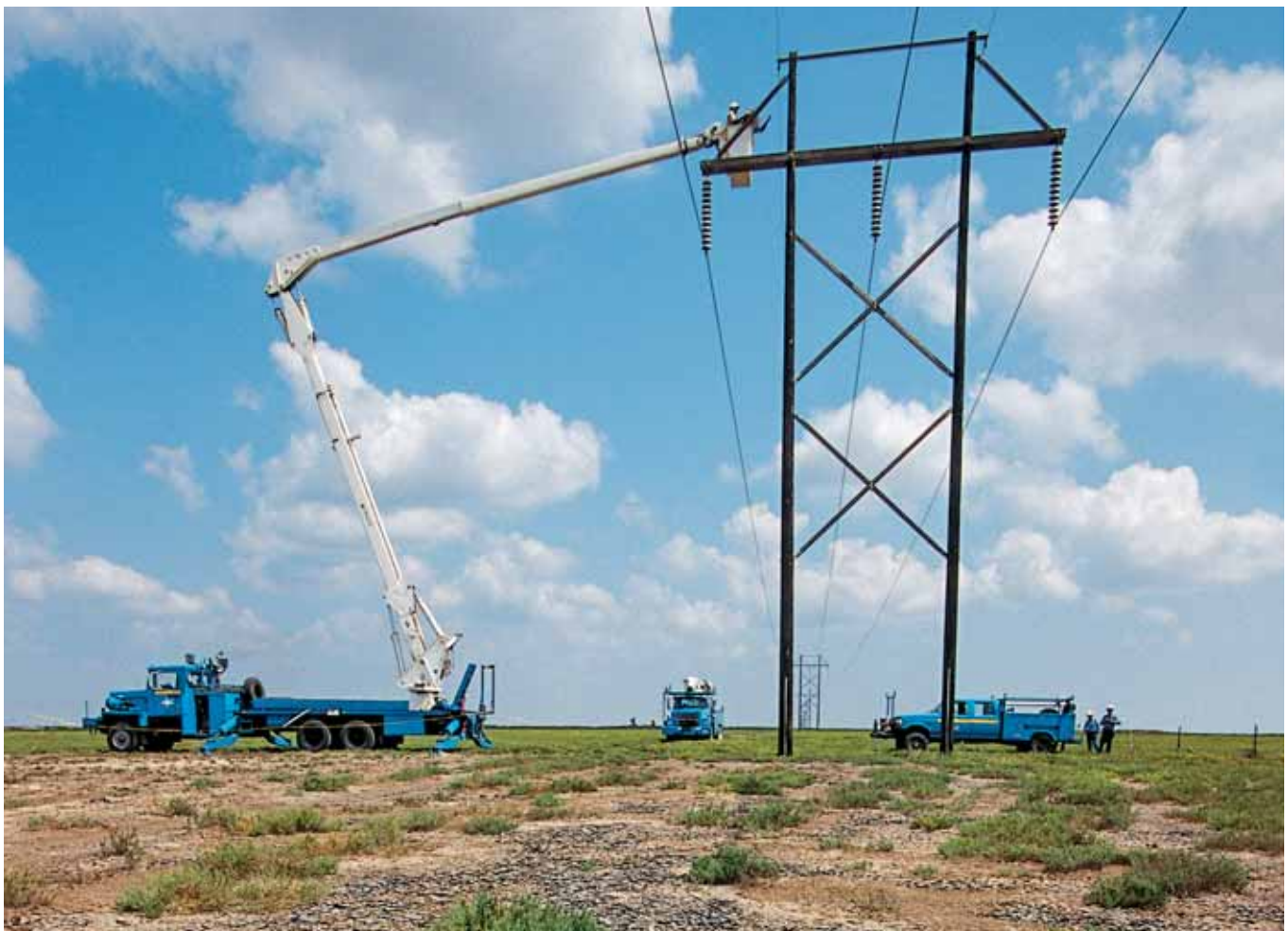
A CPL line crew works on transmission lines near Harlingen, Texas.
