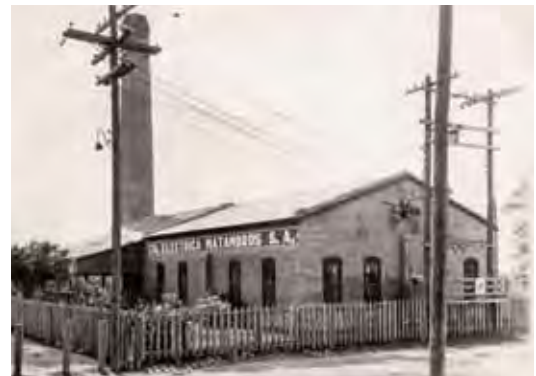
CPL's Matamoros Plant across the Rio Grande in Mexico
