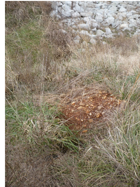
Photo #14 – rodent hole on west containment berm
