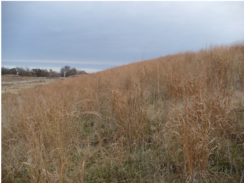
Photo #11 – final cover –west slope looking north
