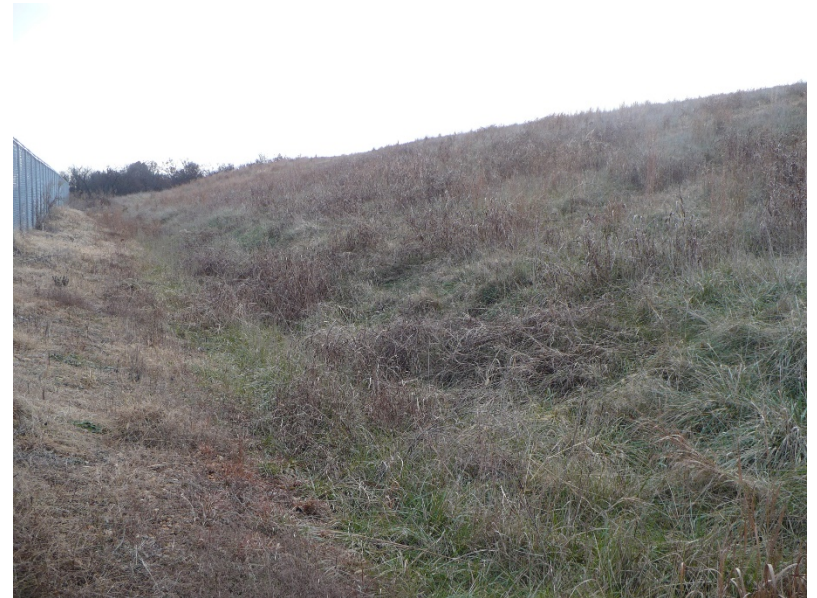
Photo #12 – final cover –north slope looking east
