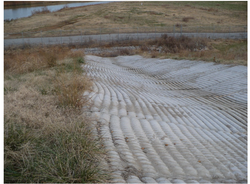
Photo #6 – North fabriform letdown channel
