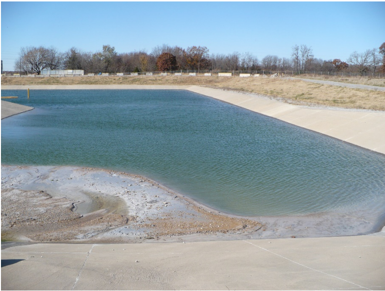
Photo #17 – North end of contact water pond
