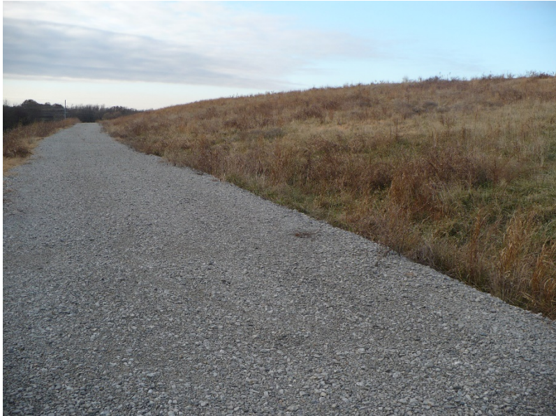
Photo #9 – final cover –east slope looking south
