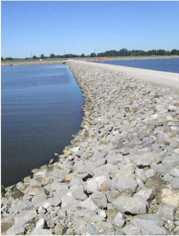
Photo #1 – interior slope of north Clearwater pond
