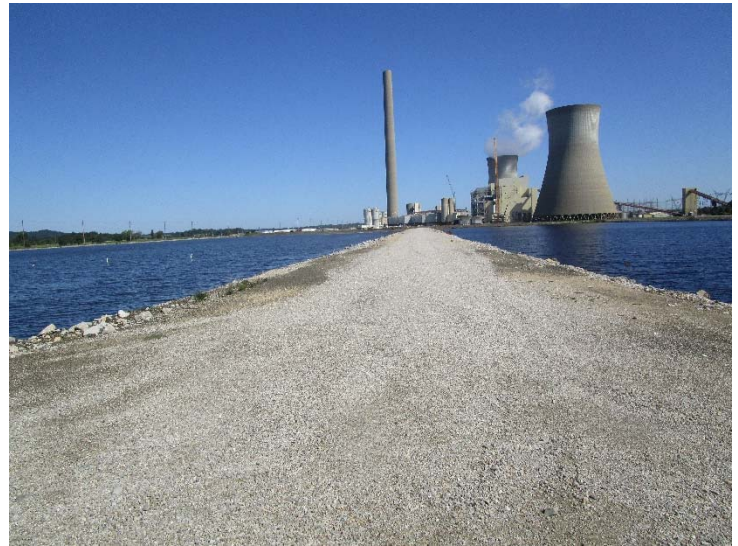
Photo #6W– splitter dike between ash ponds
