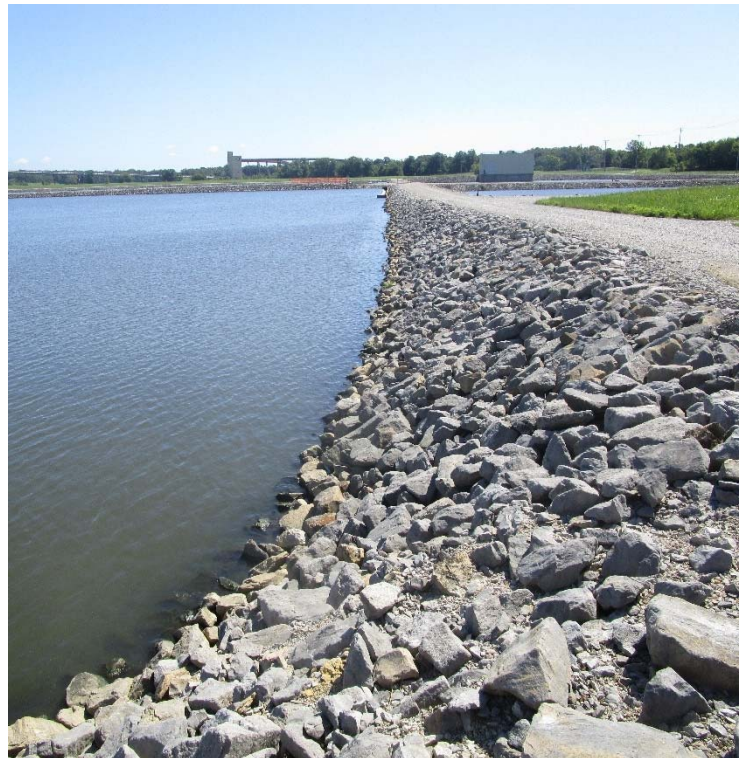
Photo #4WW – interior south slope Of West WW pond
