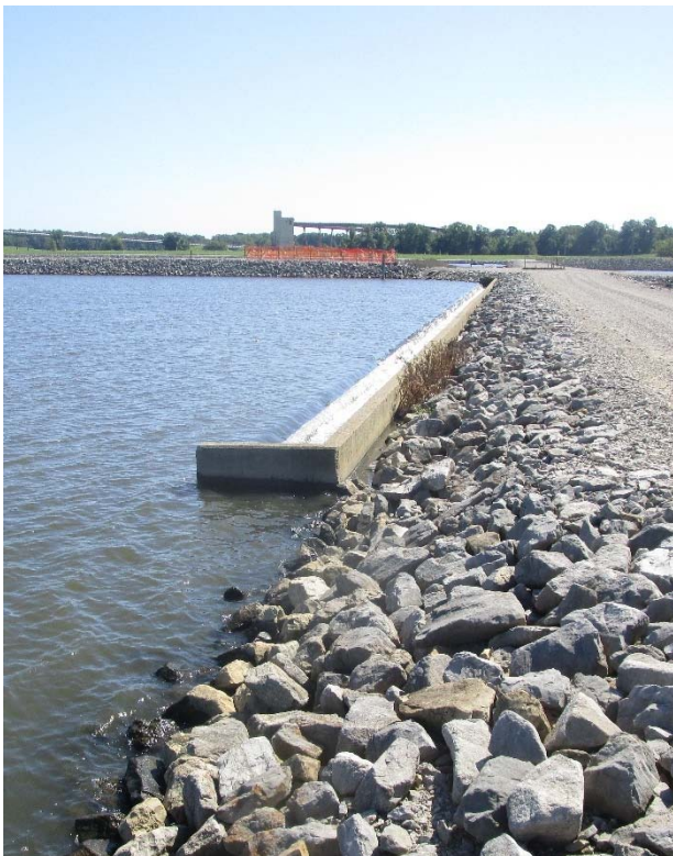
Photo #3WW – operating discharge structure in West WW pond
