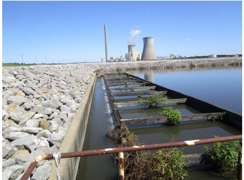
Photo #2– discharge structure at Clearwater pond
