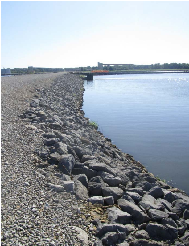
Photo #1WW – interior north slope of West WW pond
