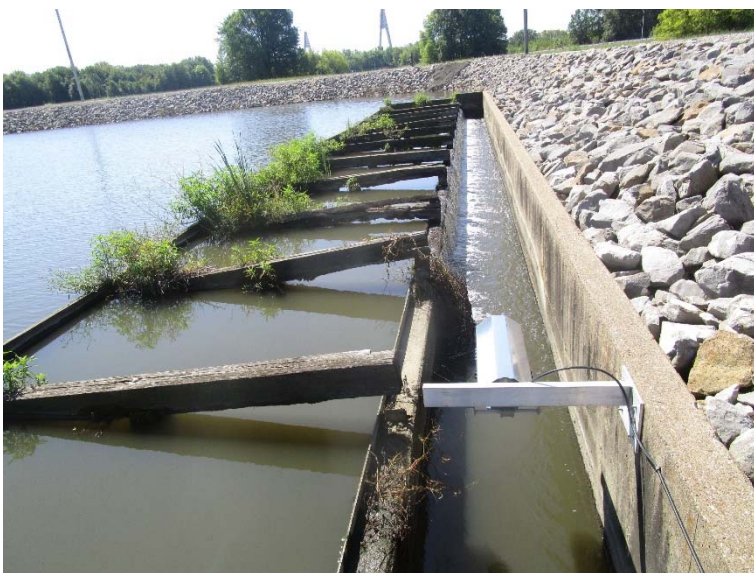
Photo #4 – discharge structure at Clearwater pond
