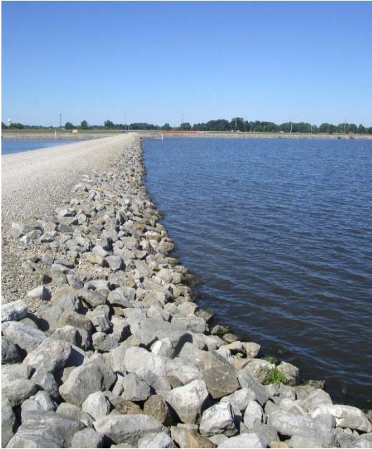
Photo #5WW – interior north slope of East WW pond
