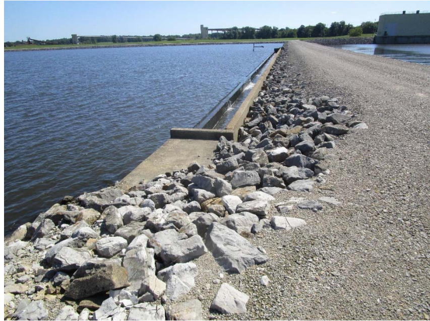
Photo #6WW– discharge weir structure at East WW pond
