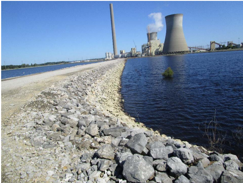
Photo #1E –Interior West Slope of East ash pond
