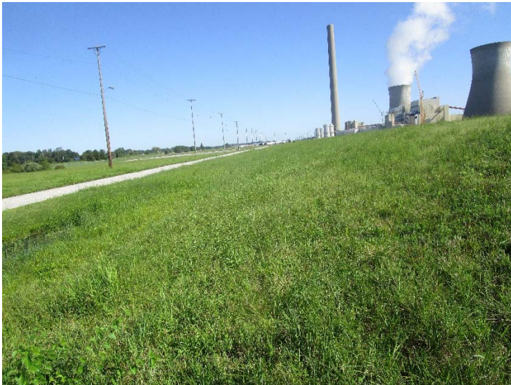
Photo #3W – toe of west dike
