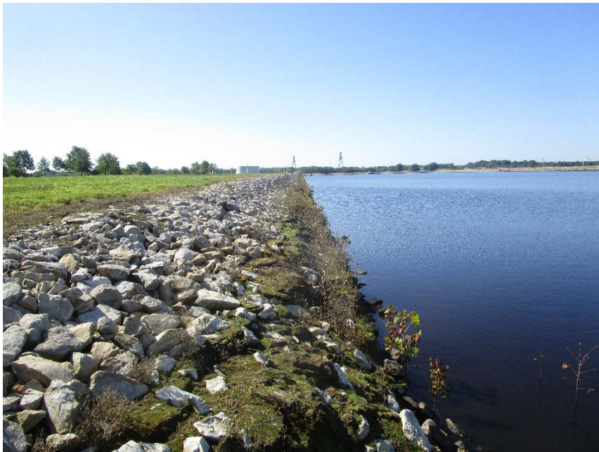
Photo #3E – Interior of east slope and ash pond
