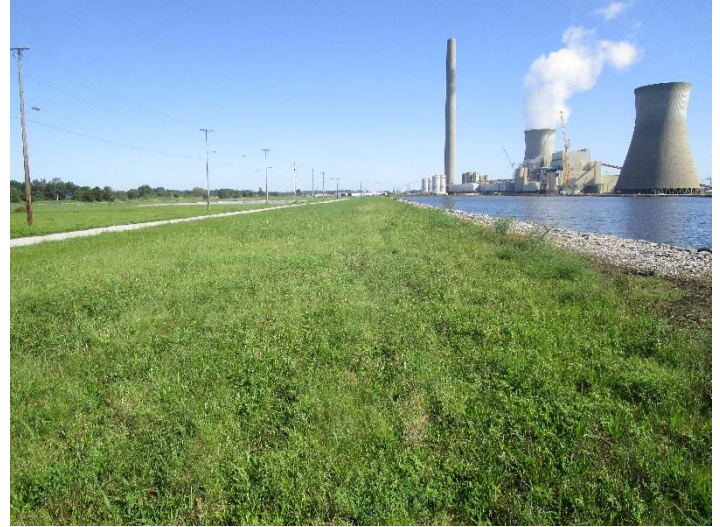
Photo #2W – crest of west dike
