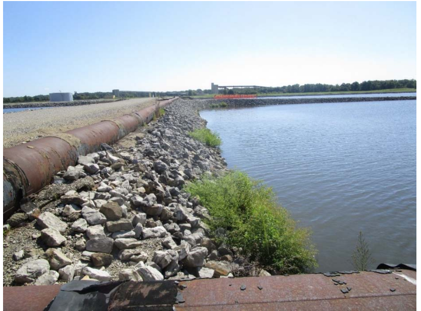
Photo #2WW– interior north slope of West WW pond
