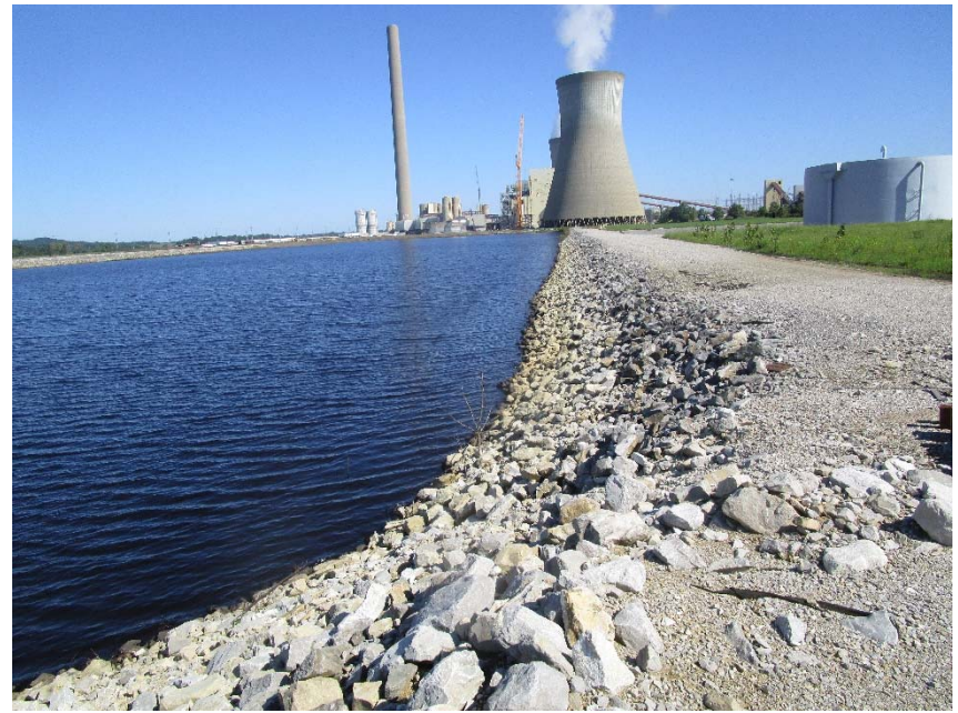
Photo #4E – Interior of east slope Looking North
