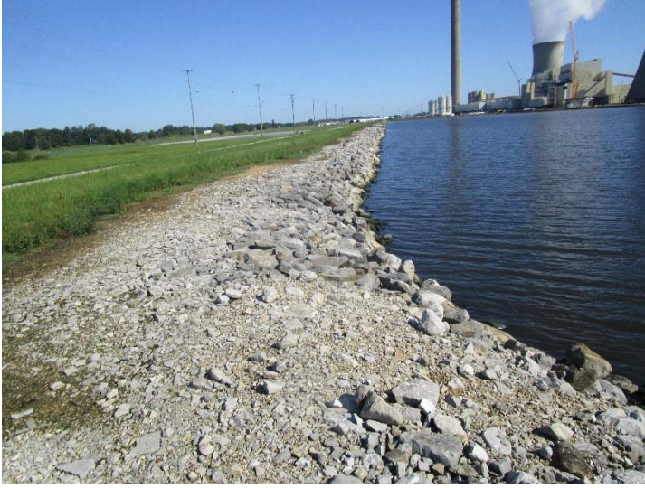
Photo #1W – interior slope of west dike
