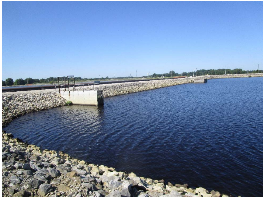
Photo #2E – South Interior Slope- Discharge Structures
