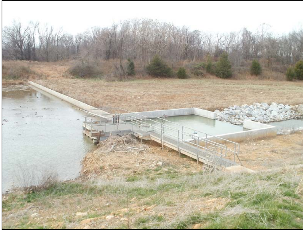
Figure 6 – Secondary Ash Pond Spillway
