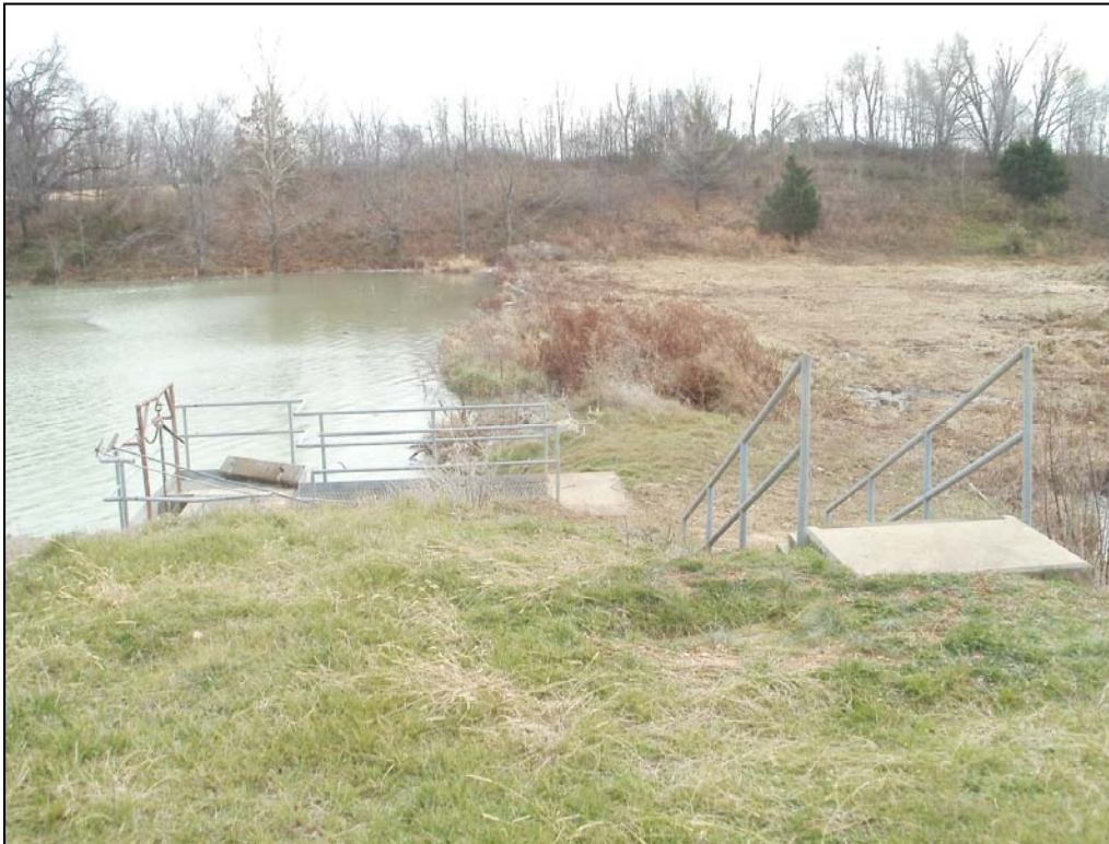
Figure 5 – Primary Ash Pond Spillway
