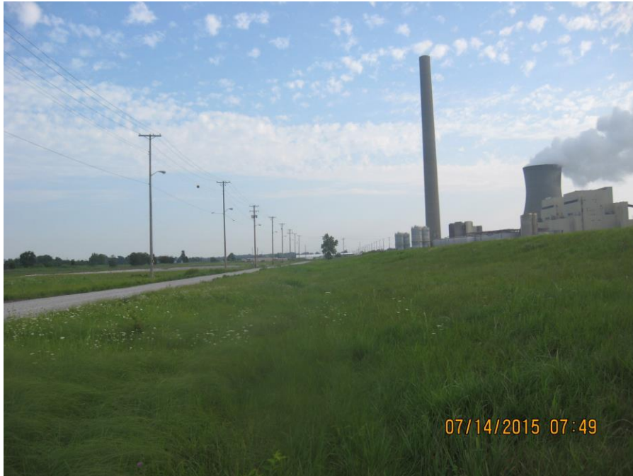
Photo 1: West Bottom Ash Pond, west dike: exterior slope (facing north).
