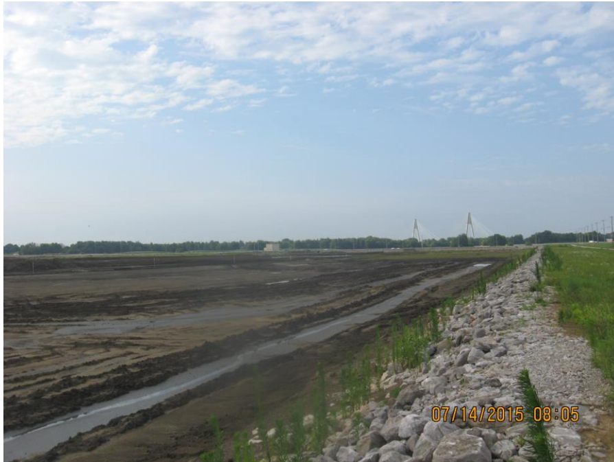
Photo 7: West Bottom Ash Pond, west dike: bottom ash pond interior.
