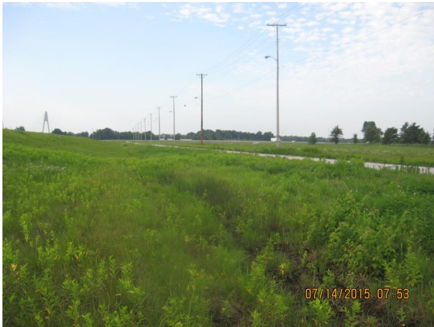
Photo 2: West Bottom Ash Pond, west dike: exterior slope (facing south).
