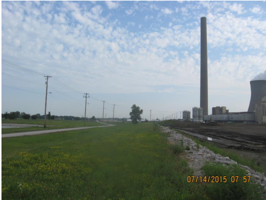
Photo 5: West Bottom Ash Pond, west dike: crest and interior slope (facing north).
