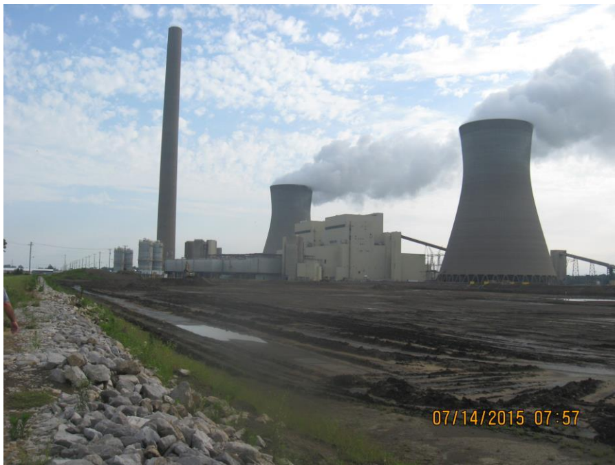
Photo 6: West Bottom Ash Pond, west dike: bottom ash pond interior.
