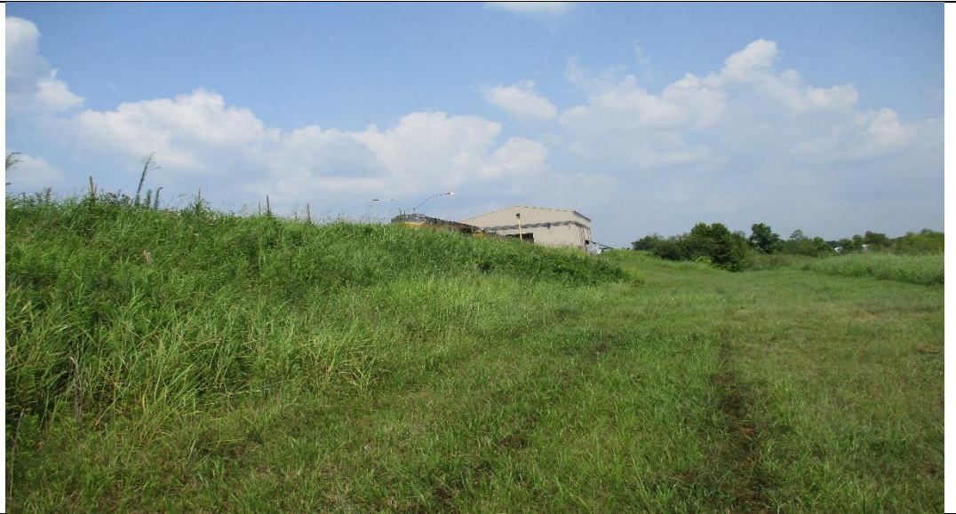
PHOTO #10 Upstream north slope (looking east).
