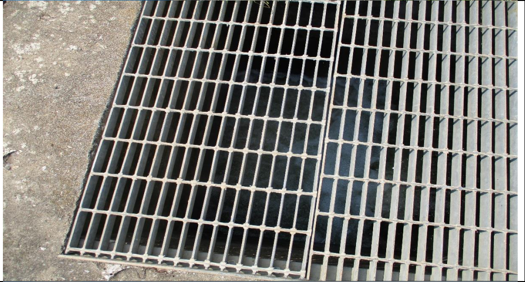
PHOTO #8 Interior of the discharge structure.
