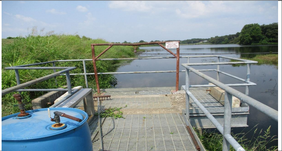
PHOTO #7 Overflow discharge structure.
