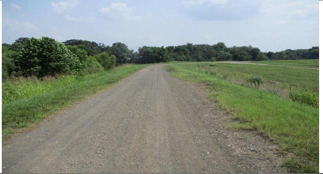
PHOTO #12 Crest of the dam (looking south).
