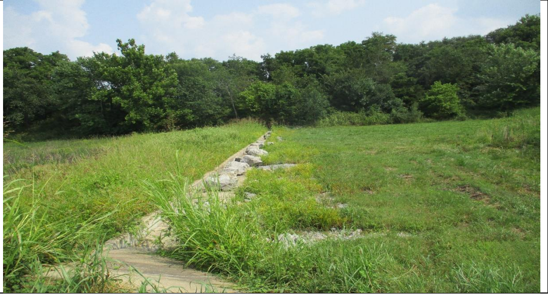
PHOTO #9 Emergency spillway concrete sill.
