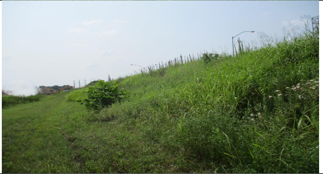
PHOTO #11 Upstream north slope (looking west).
