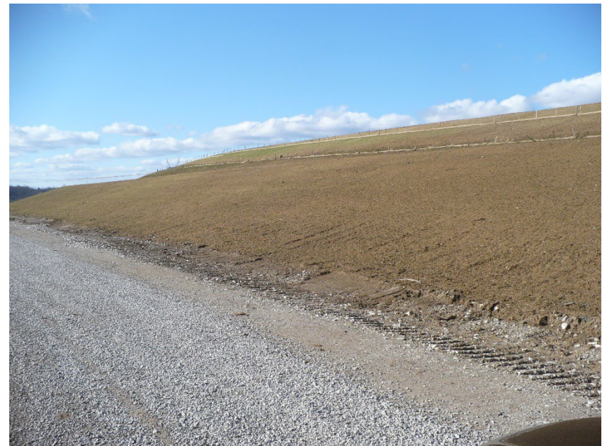
Photo #12 – New cap/cover along 950 bench
