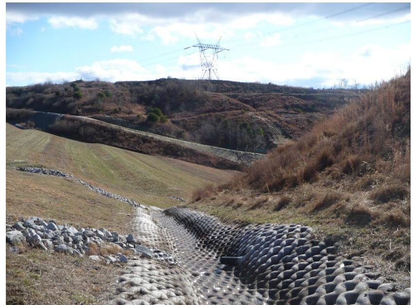
Photo #8 – South valley perimeter ditch- right abutment
