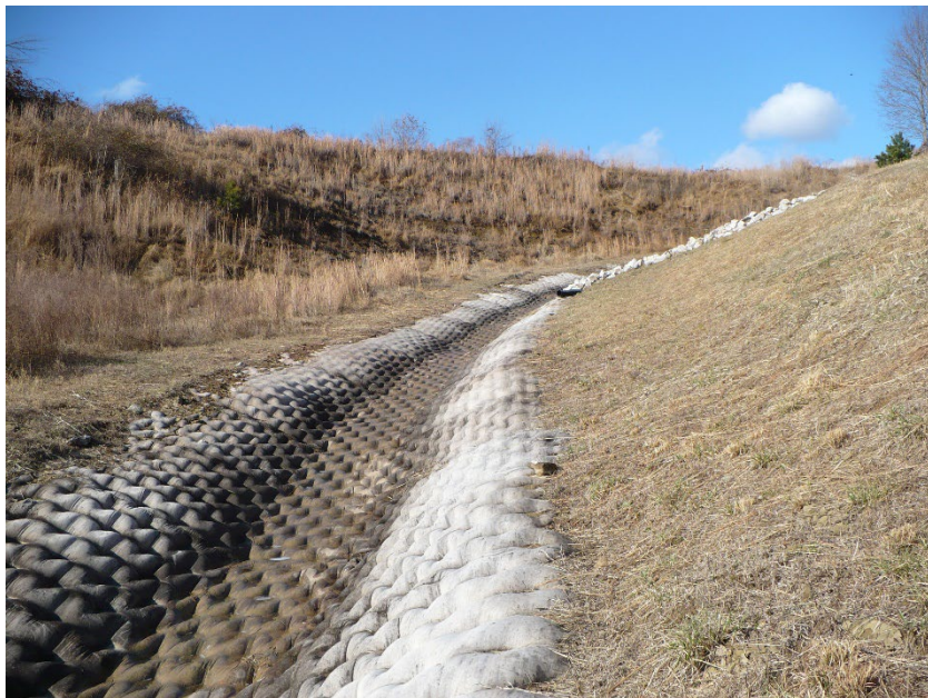
Photo #7 – South valley perimeter ditch-right abutment
