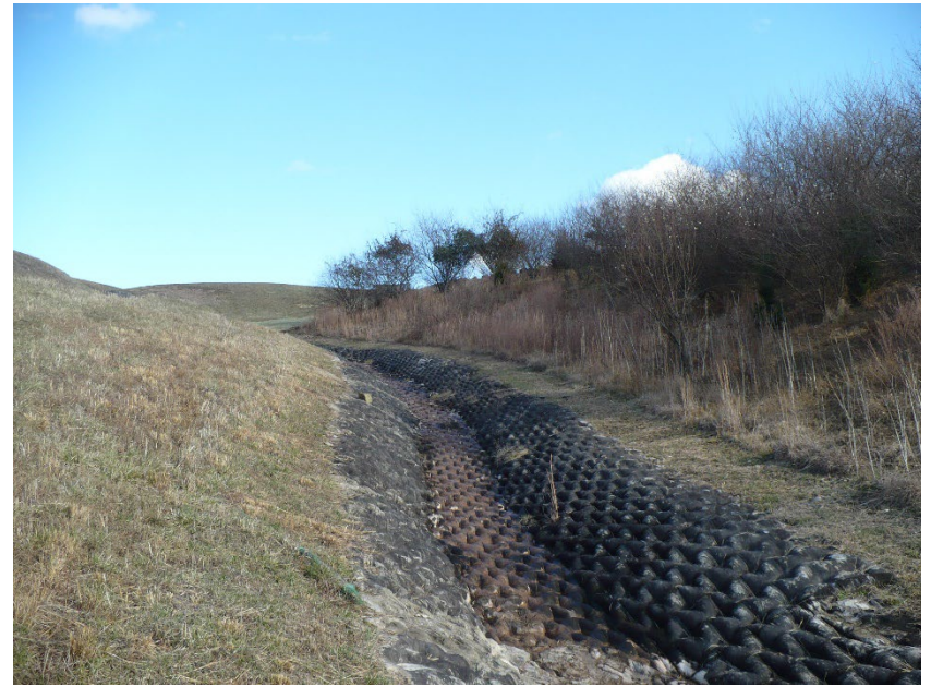
Photo #10 – South valley perimeter ditch-left abutment
