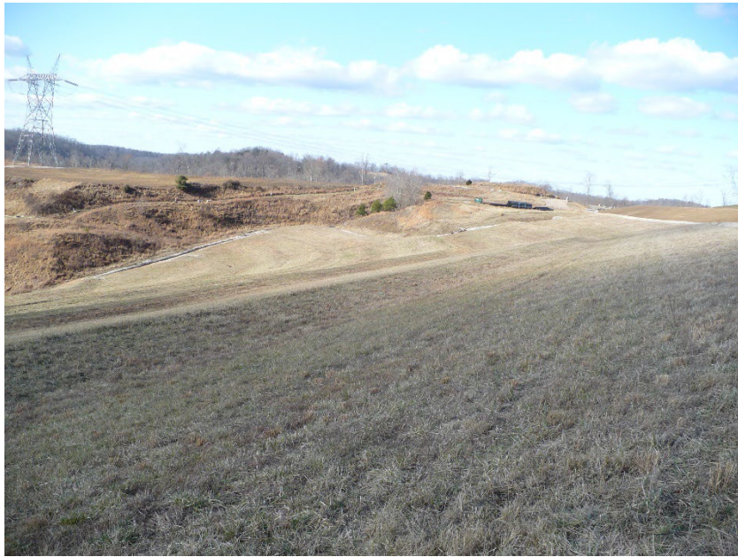
Photo #5 –covered South slope-looking north
