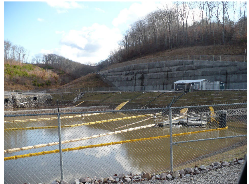
Photo #16 – Soil nail wall and sediment pond-North Valley
