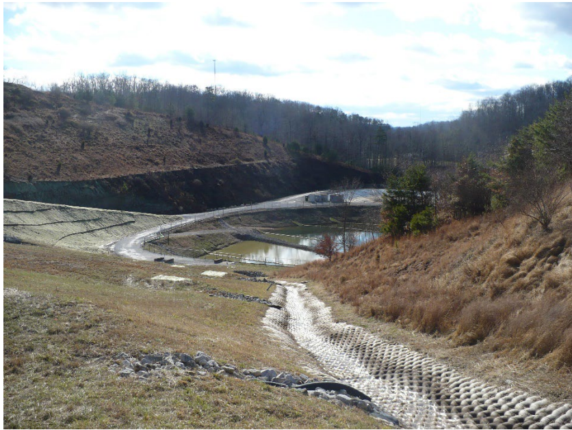
Photo #9 – South valley perimeter ditch-right abutment
