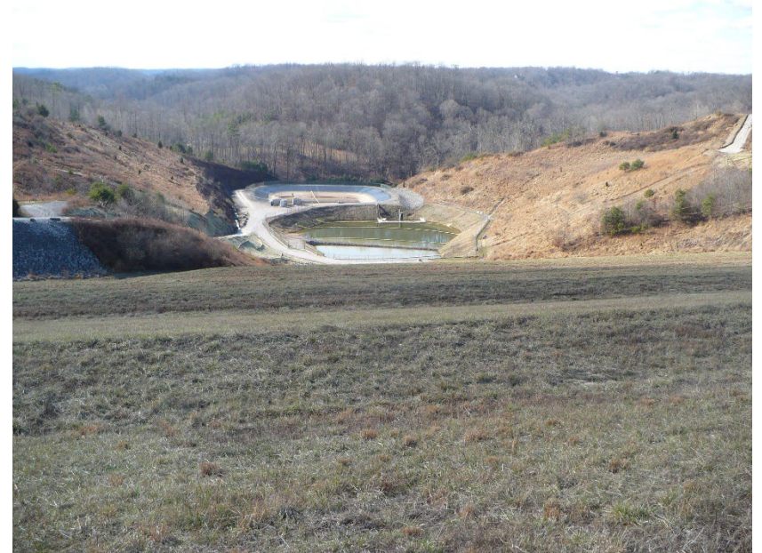
Photo #4 – closed slope of South Valley and ponds
