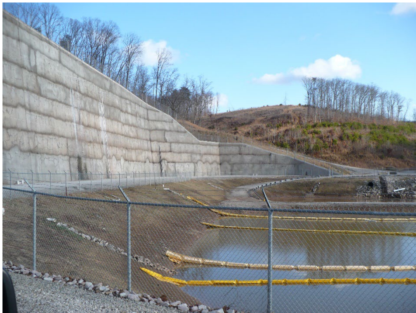
Photo #15 – Soil nail wall and sediment pond –North Valley
