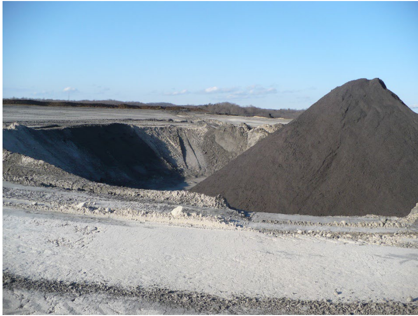
Photo #1 – chimney drain in active area
