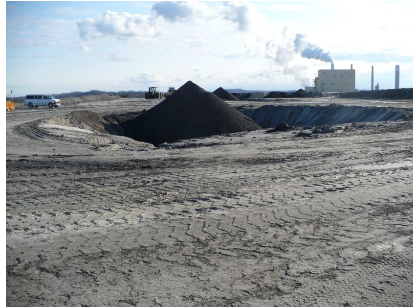
Photo #2 – chimney drain and active area
