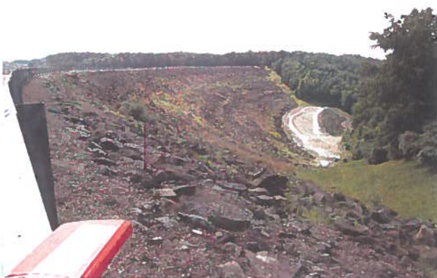
Photo 5 – Typical view showing good conditions of the right groin.
