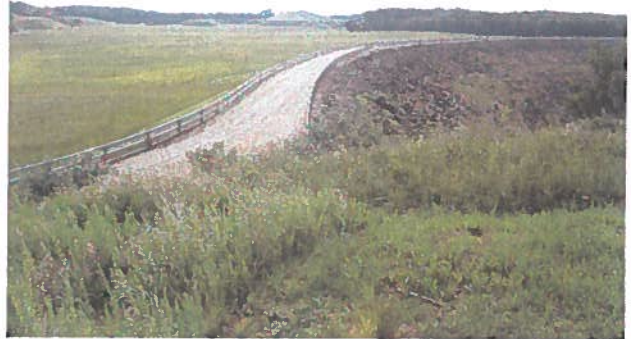
Photo 2 – Typical view showing good conditions of crest and a partial view of the capped covered pond area showing good vegetative control and maintenance.
