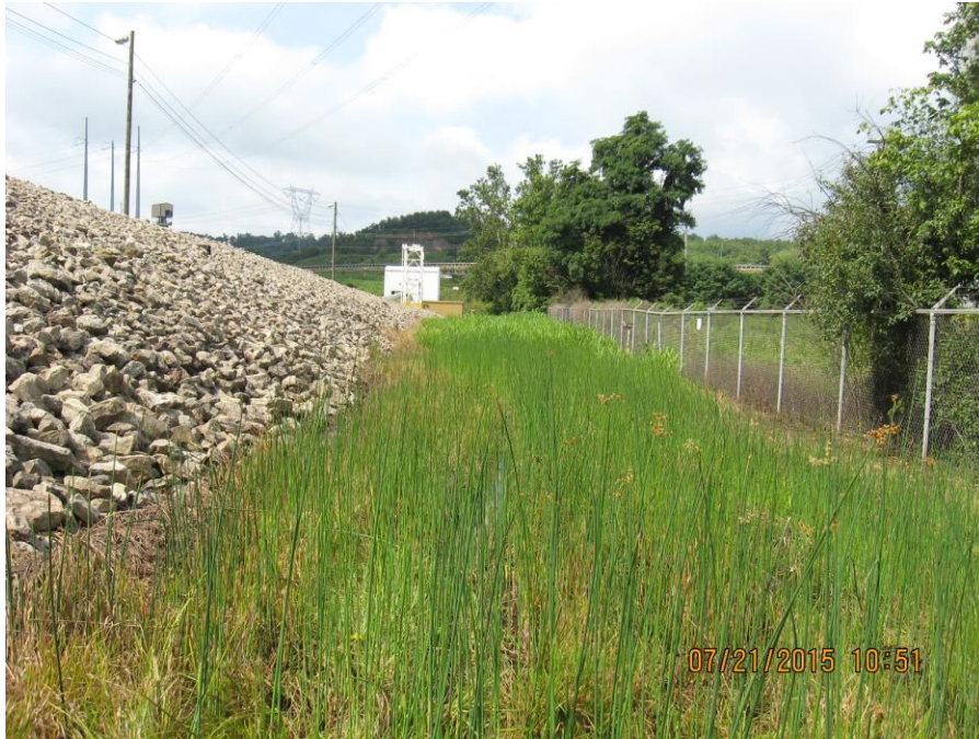
Photo 15: Bottom Ash Ponds, north dike: exterior slope.
