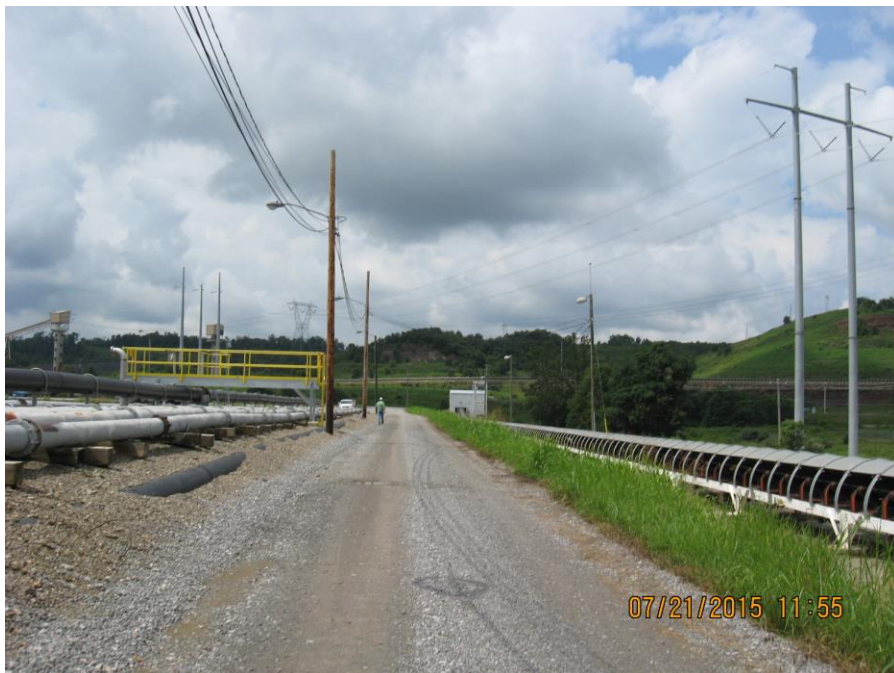
Photo 52: East Bottom Ash Pond, north dike.
