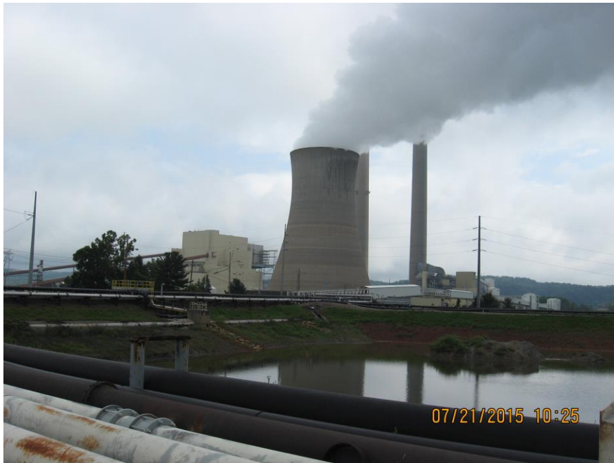
Photo 4: East Bottom Ash Pond, north/east dikes.
