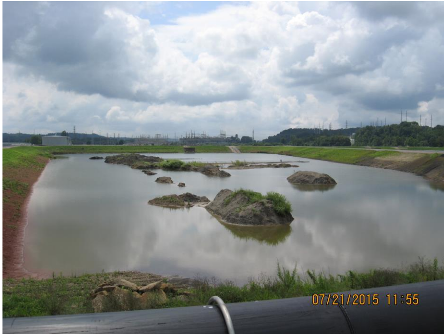
Photo 53: East Bottom Ash Pond.
