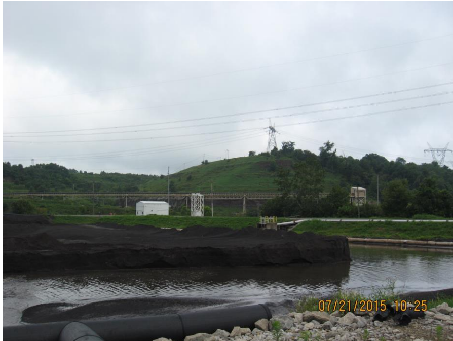
Photo 1: West Bottom Ash Pond, north dike.
