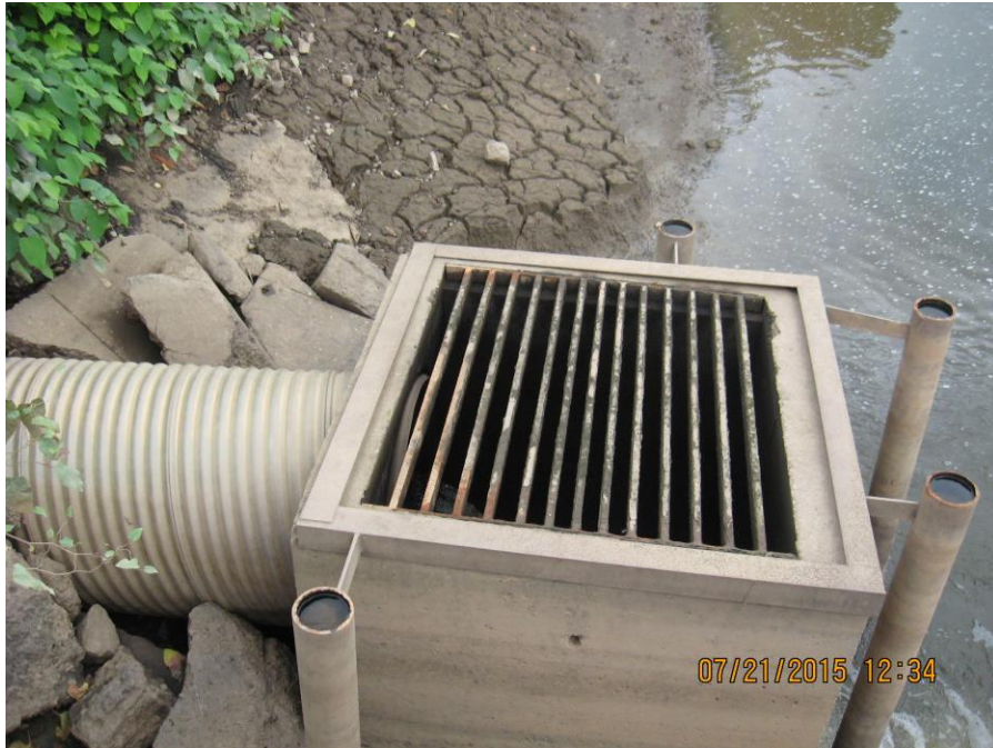
Photo 61: Ohio River outlet structure.
