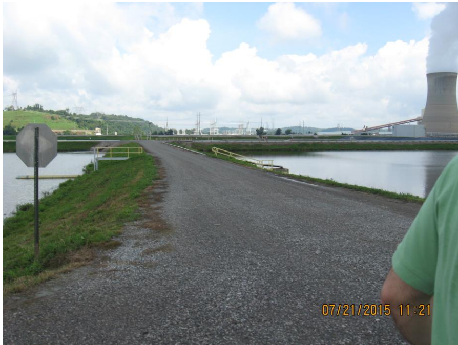
Photo 32: Reclaim Water Pond, east dike.
