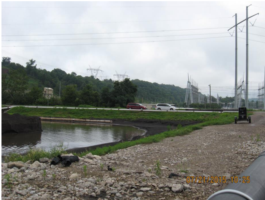
Photo 2: West Bottom Ash Pond, north dike.
