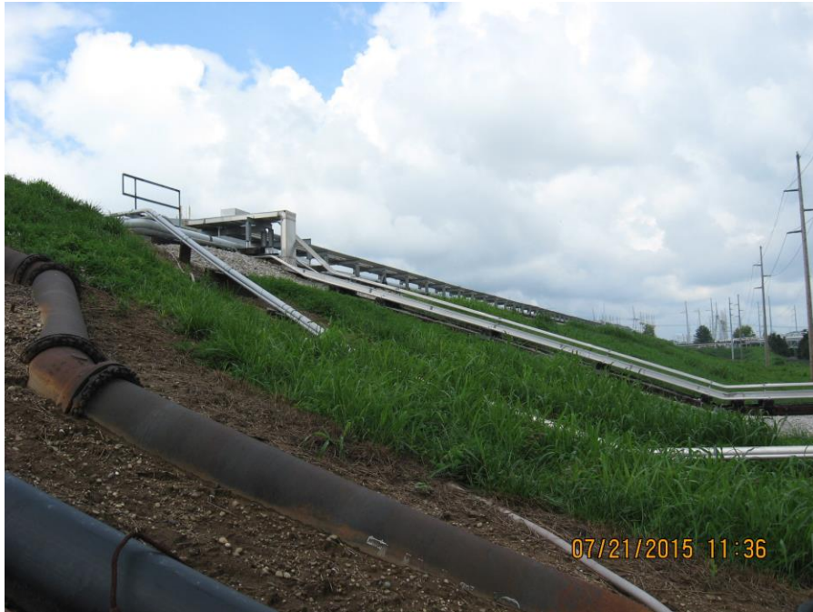
Photo 43: East Wastewater Pond, east dike: piping along exterior slope.
