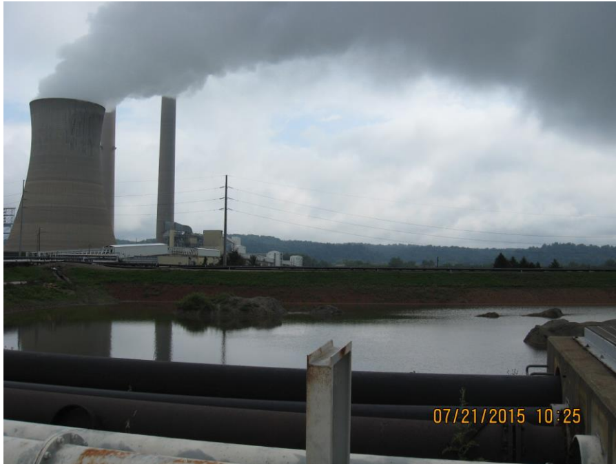
Photo 5: East Bottom Ash Pond, north/east dikes.
