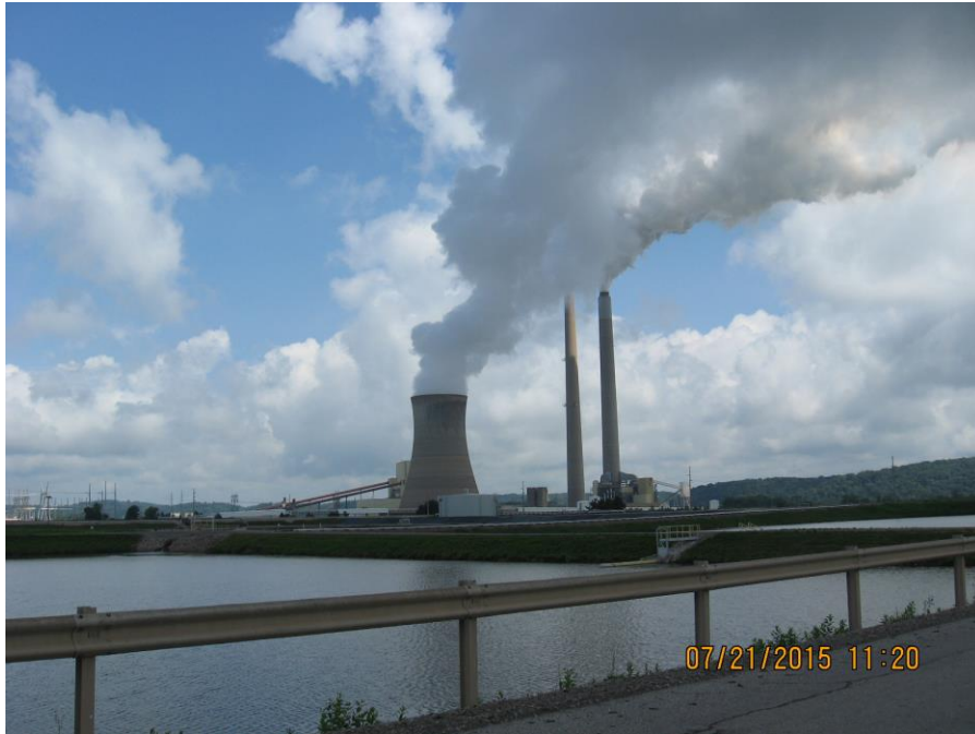
Photo 31: Reclaim Water Pond, east dike.
