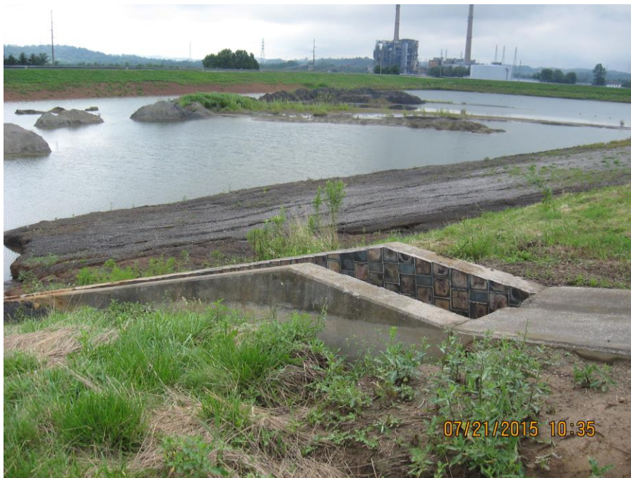
Photo 10: East Bottom Ash Pond: inlet structure.
