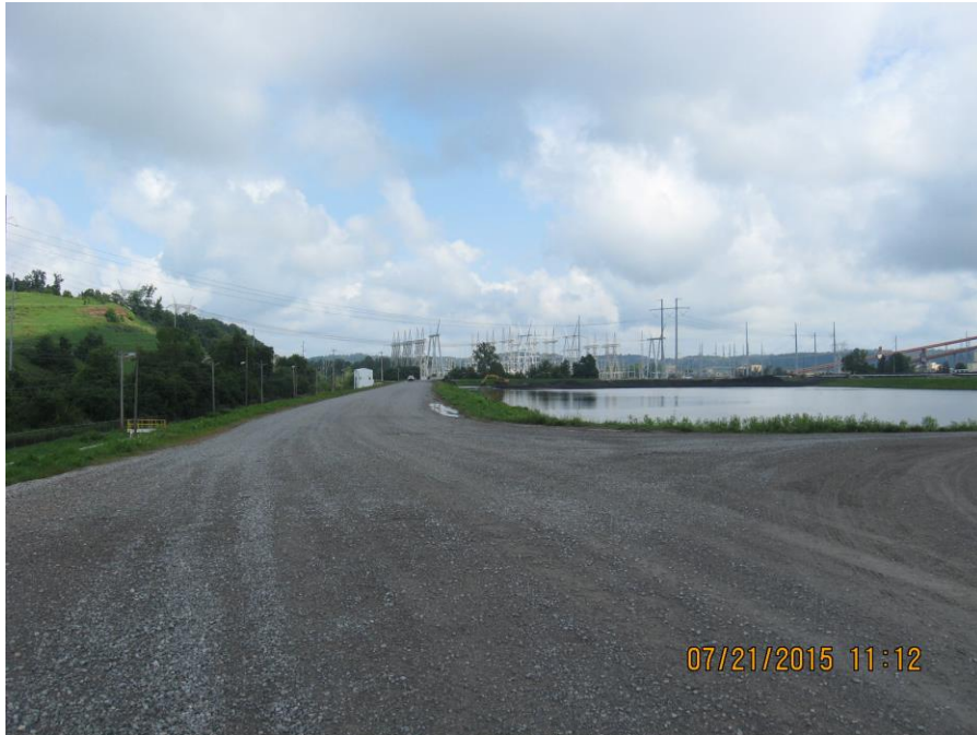
Photo 25: West Bottom Ash Pond, west dike.
