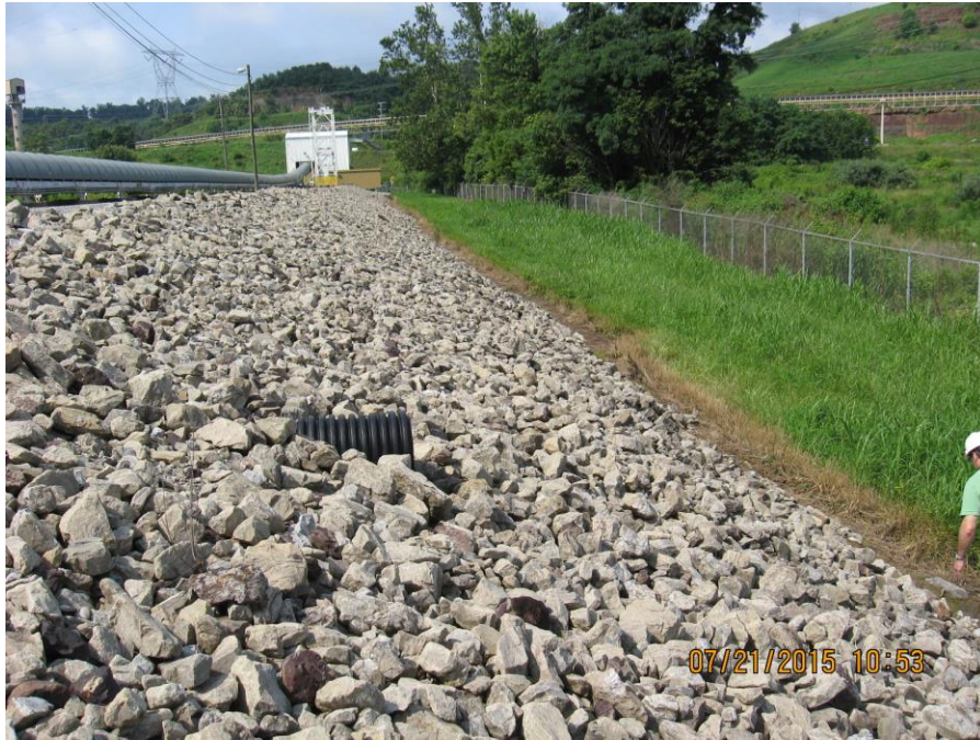
Photo 19: Bottom Ash Ponds, north dike: exterior slope.
