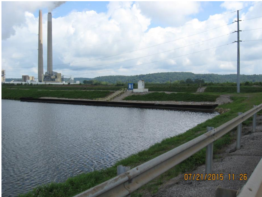
Photo 34: Clearwater Pond, outlet weir.
