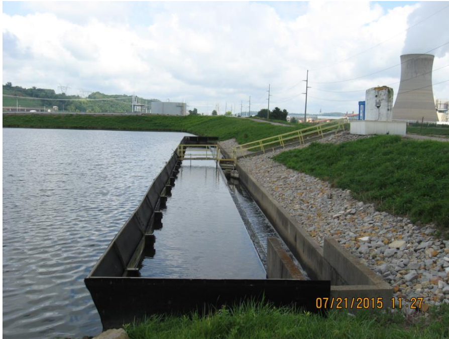
Photo 35: Clearwater Pond, outlet weir.
