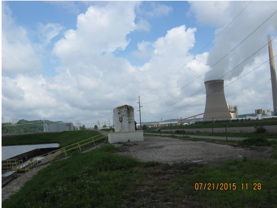
Photo 39: Clearwater Pond, east dike.
