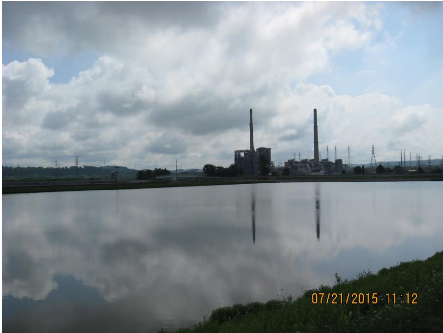
Photo 27: West Waste Water Pond, east dike.
