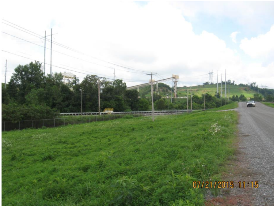
Photo 29: West Waste Water Pond, west dike.
