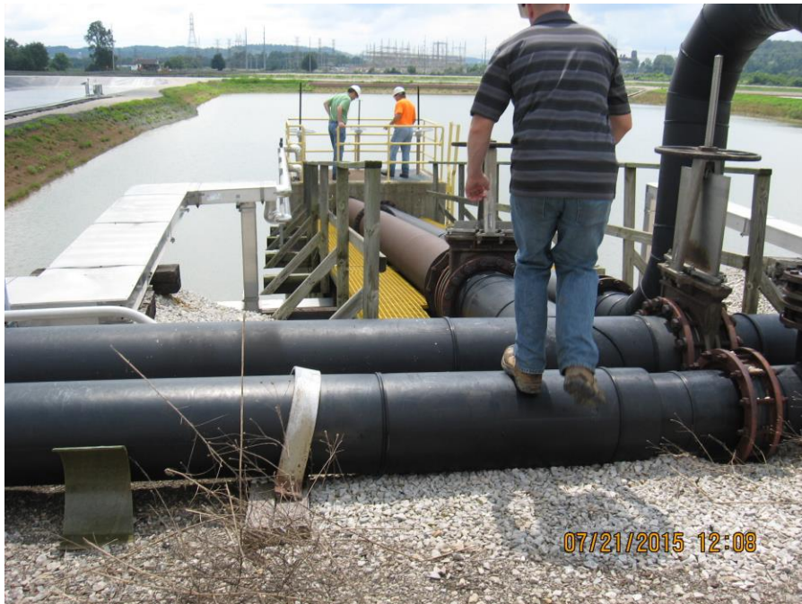
Photo 56: East Waste Water Pond: outlet structure.
