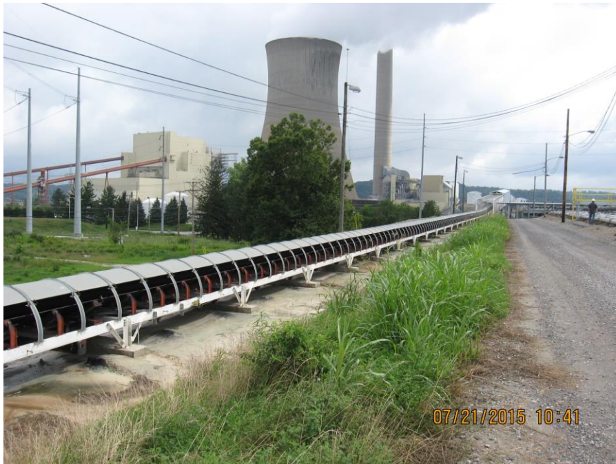
Photo 12: Bottom Ash Ponds, north dike: gypsum conveyor.
