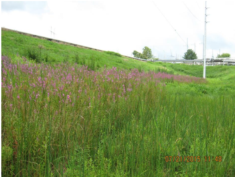
Photo 48: East Bottom Ash Pond, east dike: exterior slope.
