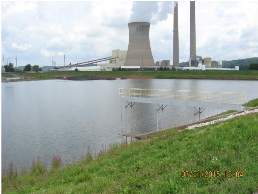
Photo 54: East Bottom Ash Pond, south dike: outlet structure.
