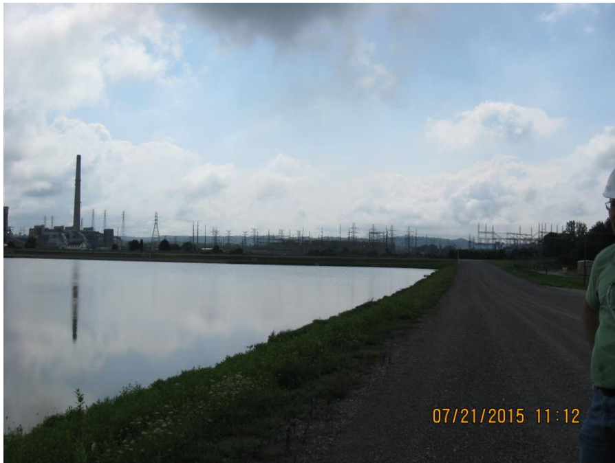
Photo 28: West Waste Water Pond, west dike.
