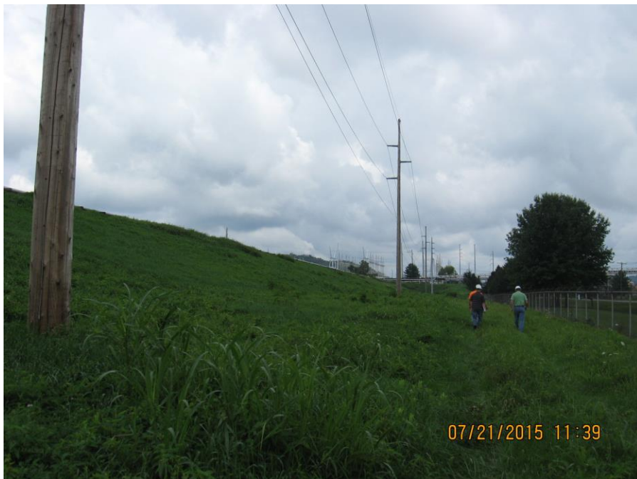
Photo 44: East Wastewater Pond, east dike.
