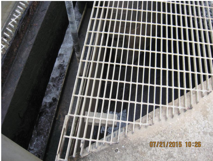
Photo 7: West Bottom Ash Pond: inlet structure sluice gate.
