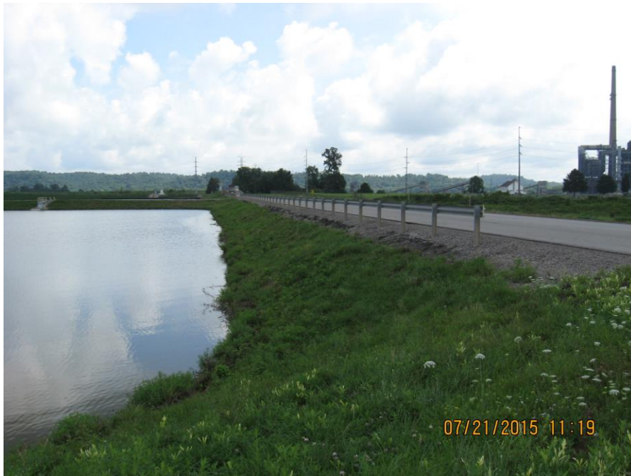
Photo 30: Reclaim Water Pond, south dike.
