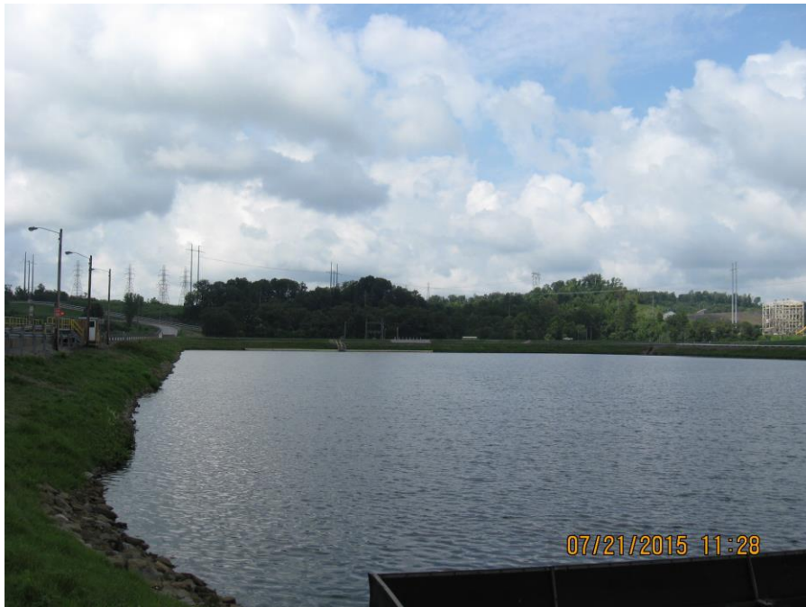
Photo 36: Clearwater Pond, west dike.
