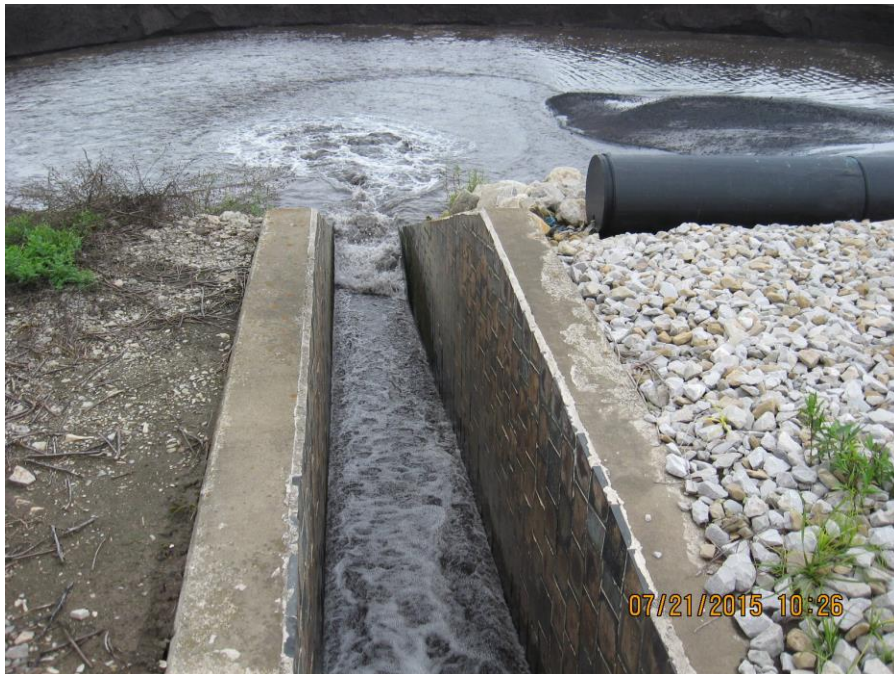
Photo 6: West Bottom Ash Pond: inlet structure.
