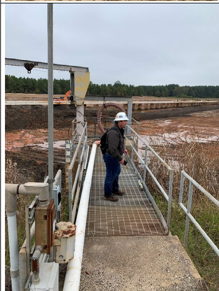
Photograph 7: East Bottom Ash Pond
