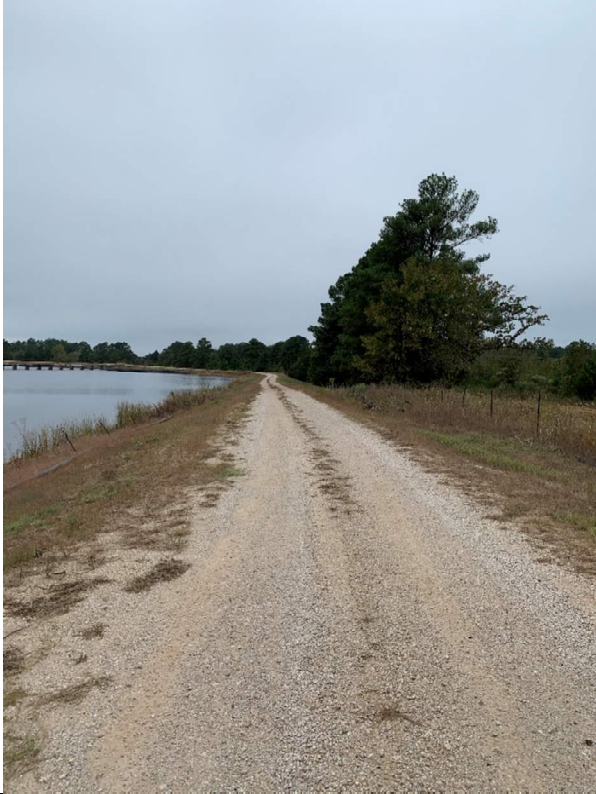
Photograph 8: West Bottom Ash Pond
