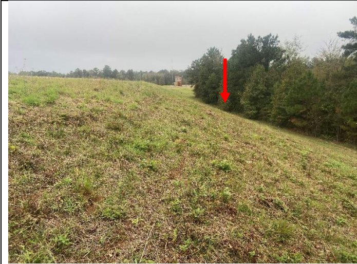
Photograph 10: West Bottom Ash Pond
