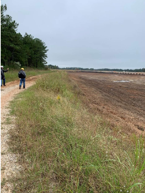
Photograph 4: East Bottom Ash Pond
