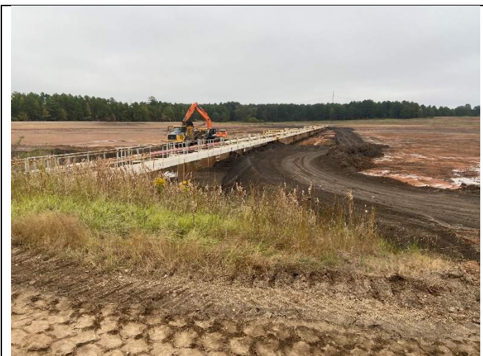
Photograph 6: East Bottom Ash Pond
