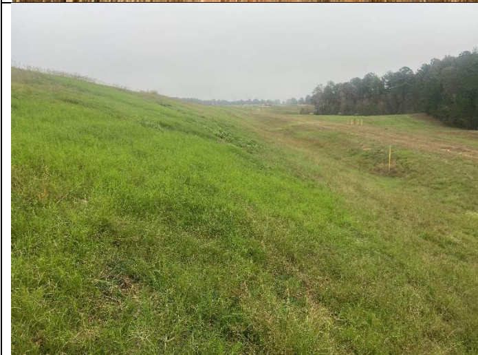
Photograph 15: West Bottom Ash Pond
