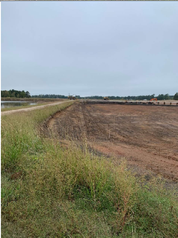
Photograph 5: East Bottom Ash Pond
