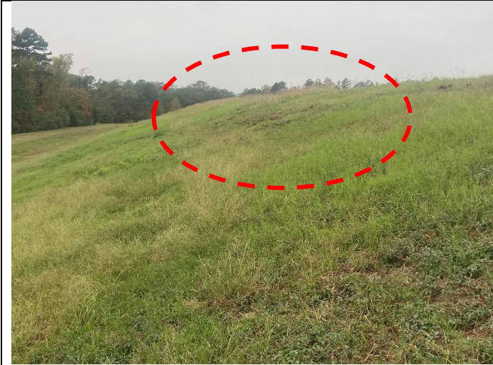
Photograph 16: West Bottom Ash Pond
