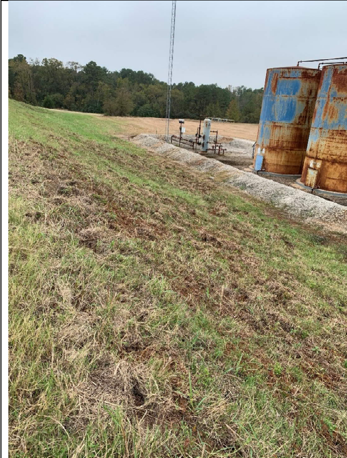
Photograph 12: West Bottom Ash Pond
