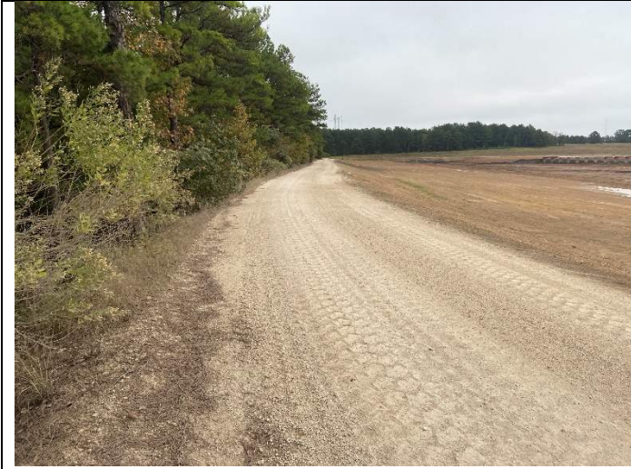
Photograph 1: East Bottom Ash Pond
