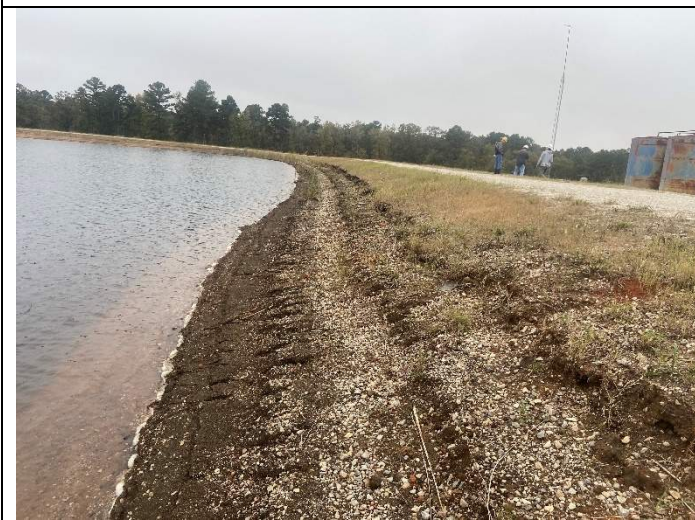
Photograph 11: West Bottom Ash Pond
