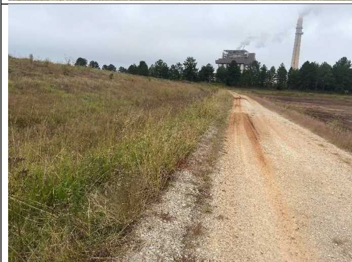
Photograph 3: East Bottom Ash Pond
