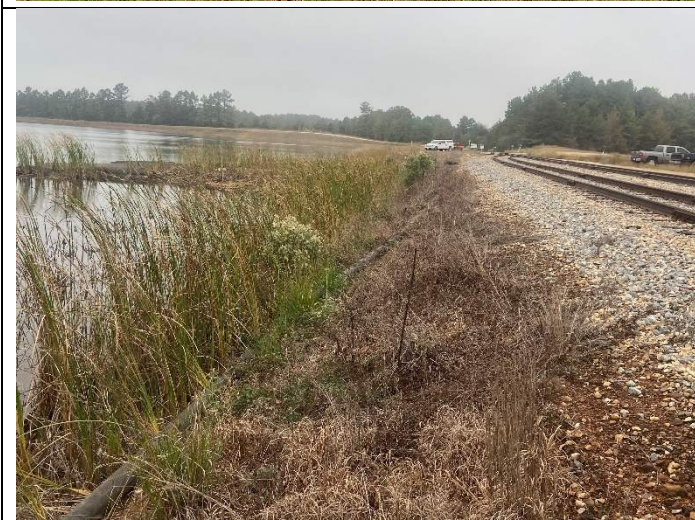
Photograph 18: West Bottom Ash Pond
