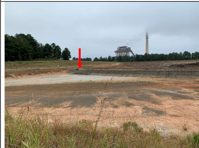
Photograph 2: East Bottom Ash Pond
