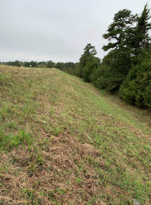
Photograph 9: West Bottom Ash Pond
