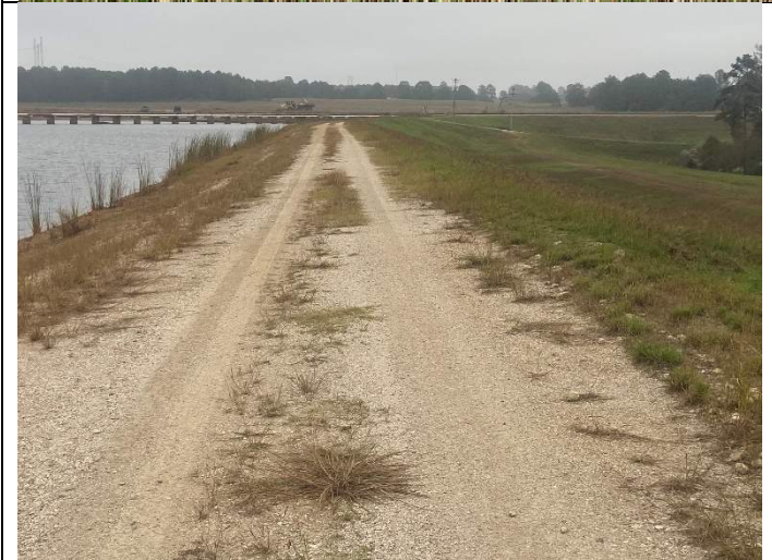
Photograph 13: West Bottom Ash Pond
