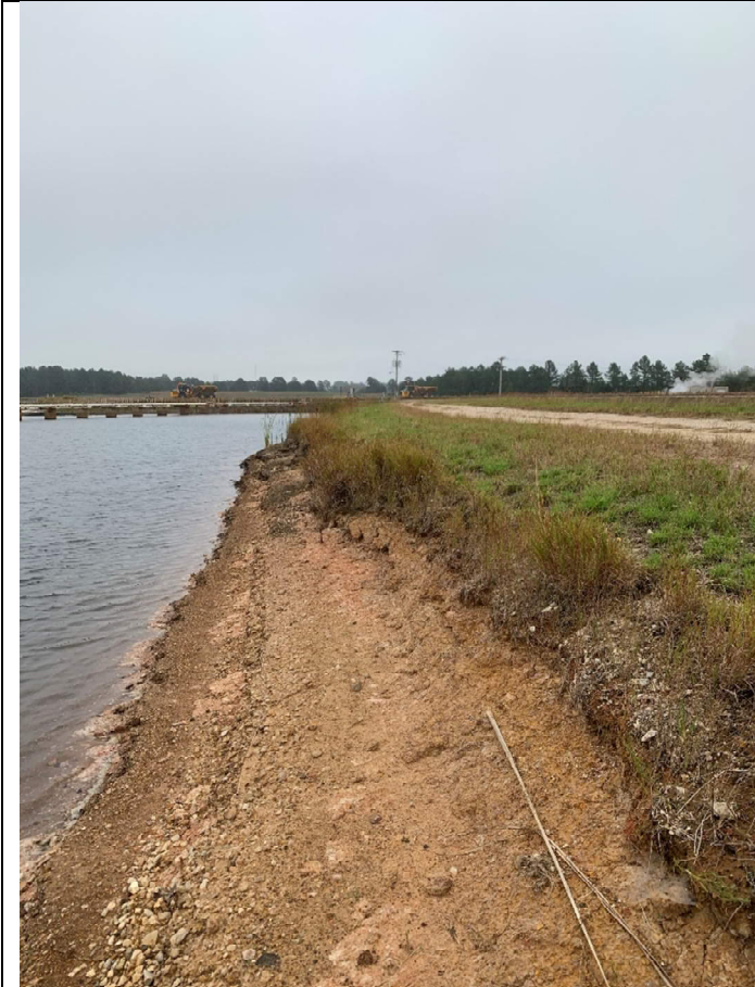
Photograph 14: West Bottom Ash Pond
