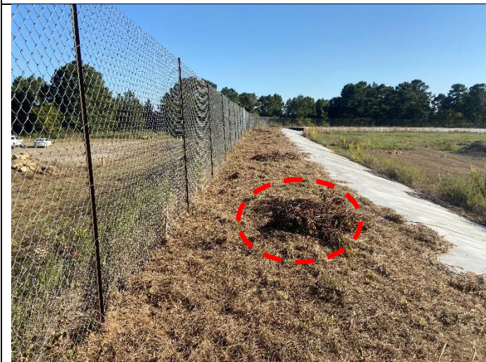
Photograph 2: Example of animal burrowing activity on the crest. East embankment, looking south.
