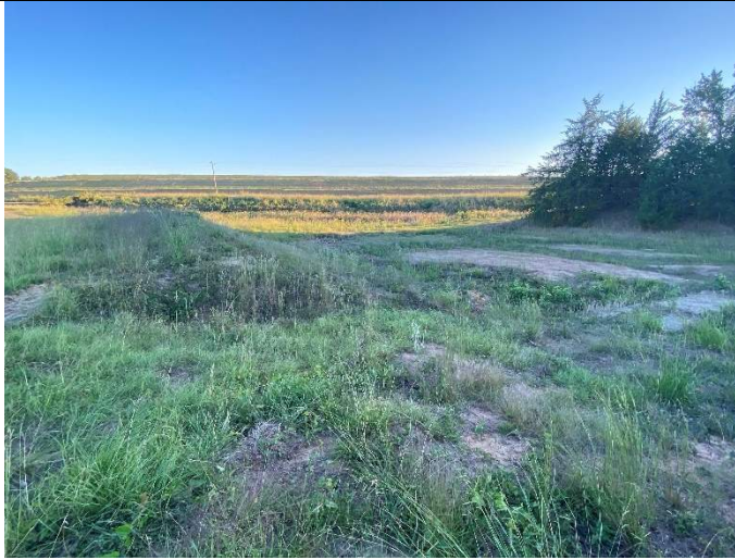
Photograph 10: View of primary emergency spillway, looking downstream, from near the overflow weir location.
