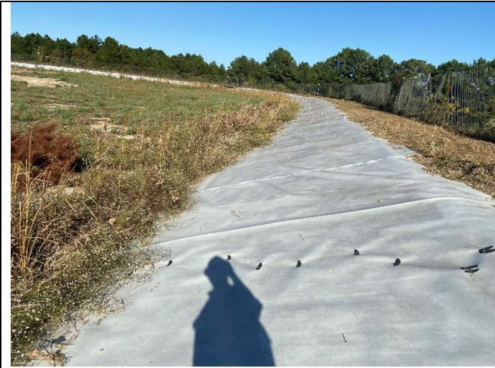
Photograph 4: Typical view of upstream slope and geosynthetic liner. East embankment, looking east.
