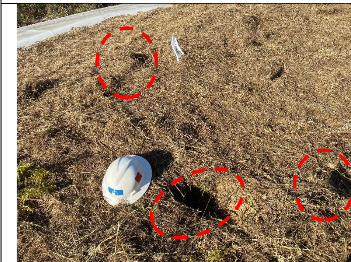
Photograph 3: Example of multiple animal burrows which were visible after the crest had been mowed.
