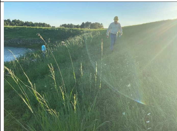
Photograph 6: Typical view of downstream slope, looking right.
