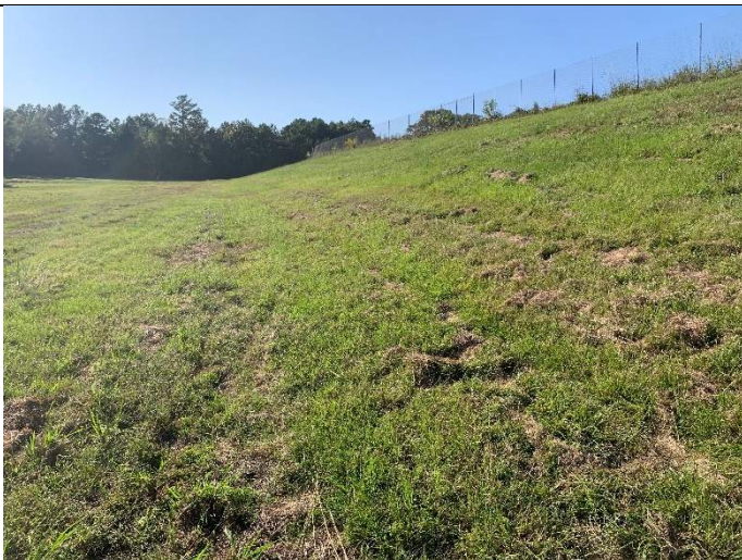
Photograph 18: Typical view of downstream slope of south embankment, looking west.
