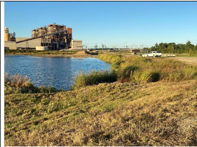
Photograph 4: Overview of upstream slope and crest, looking left, as seen from the right end of the dam.
