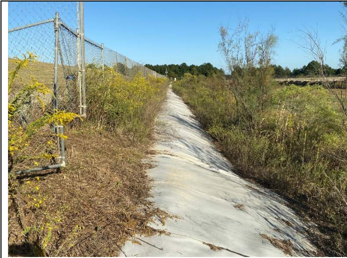
Photograph 13: Typical view of crest and upstream slope on north embankment. Note crest is overgrown with vegetation.
