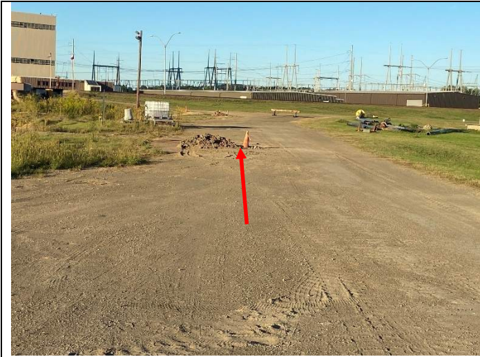
Photograph 1: View along crest, looking left. Arrow points to location of recent boring locations.
