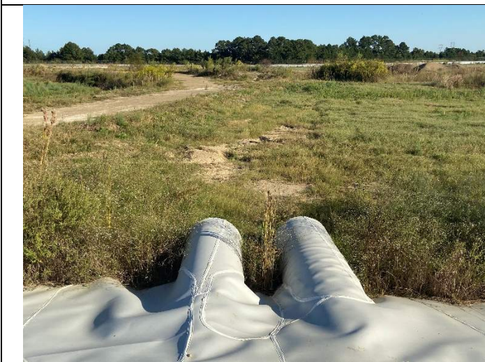
Photograph 12: View of stormwater inlet pipes entering northwest corner of pond.
