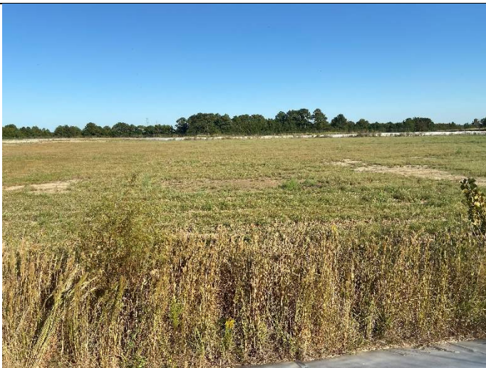
Photograph 21: View across pond, looking west from west embankment. Ash management operations appear good.
