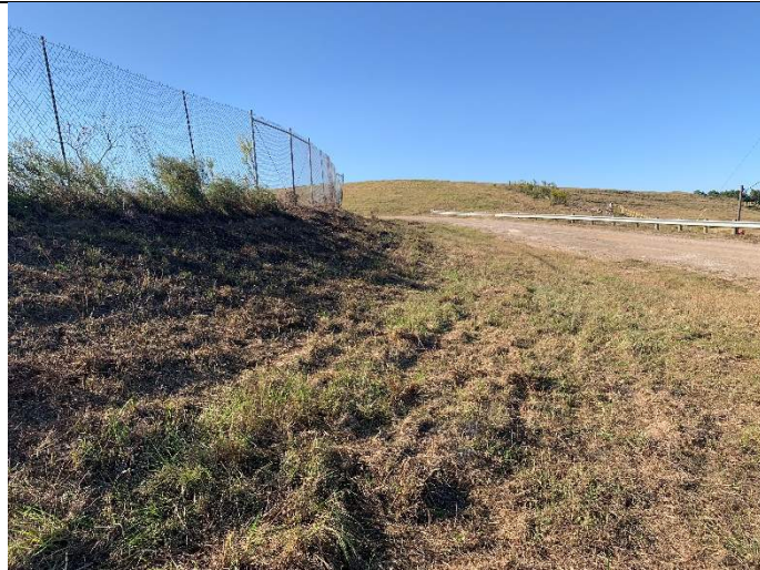
Photograph 15: Typical view of downstream slope of east embankment, looking north
