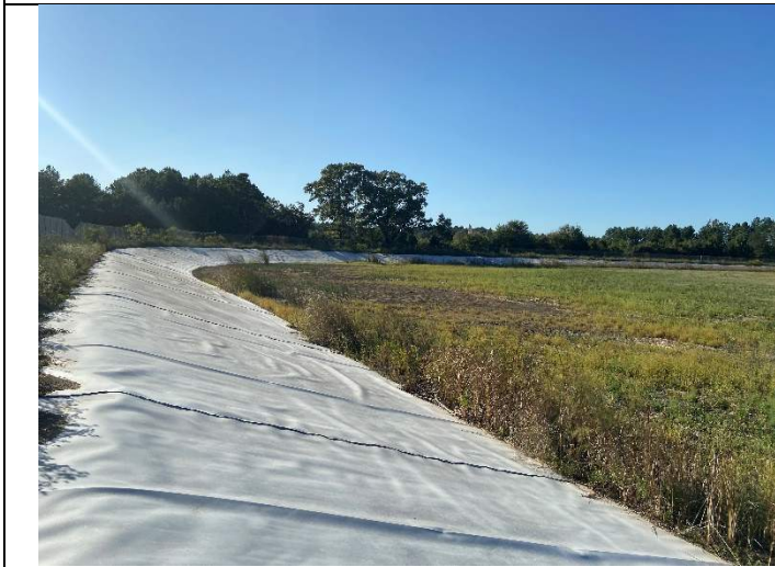
Photograph 8: View of upstream slope along south embankment, looking west.
