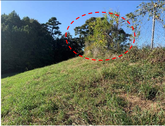
Photograph 19: View of vine vegetation growing in crest fence, as seen from downstream slope.
