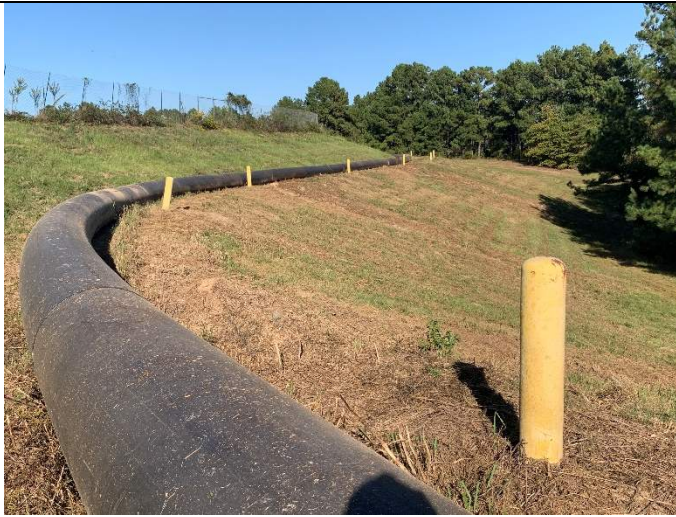
Photograph 16: Typical view of downstream slope and conveyance piping, along east embankment looking east. Note slope is well mowed.
