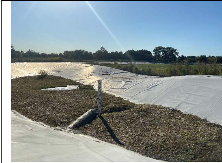
Photograph 7: View of principal spillway outlet pipe and control weir at southeast corner of pond.
