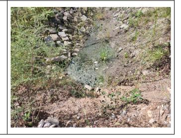
Observation 2: Minor Erosion in the temporary soil cover
