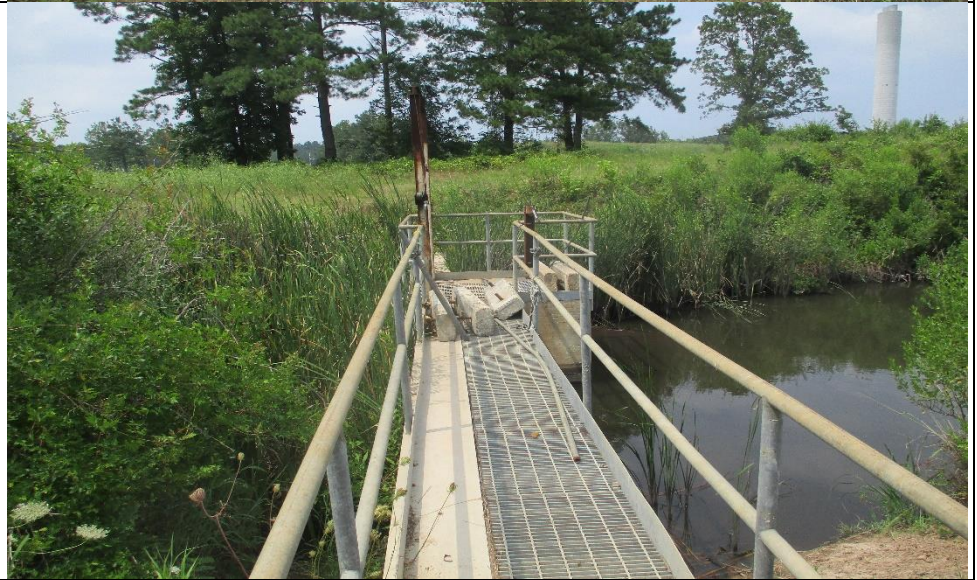
Photograph No. 14 Overflow discharge structure.
