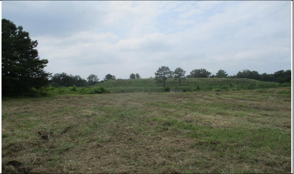
Photograph No. 12 Emergency spillway (looking north).
