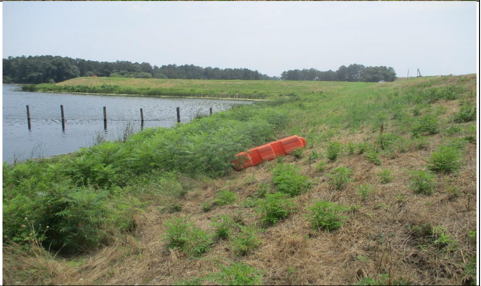
Photograph No. 5 Typical downstream slope (looking south).
