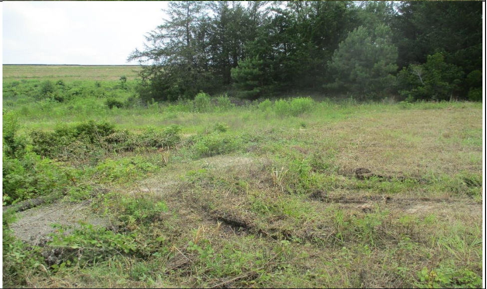
Photograph No. 11 Emergency spillway.
