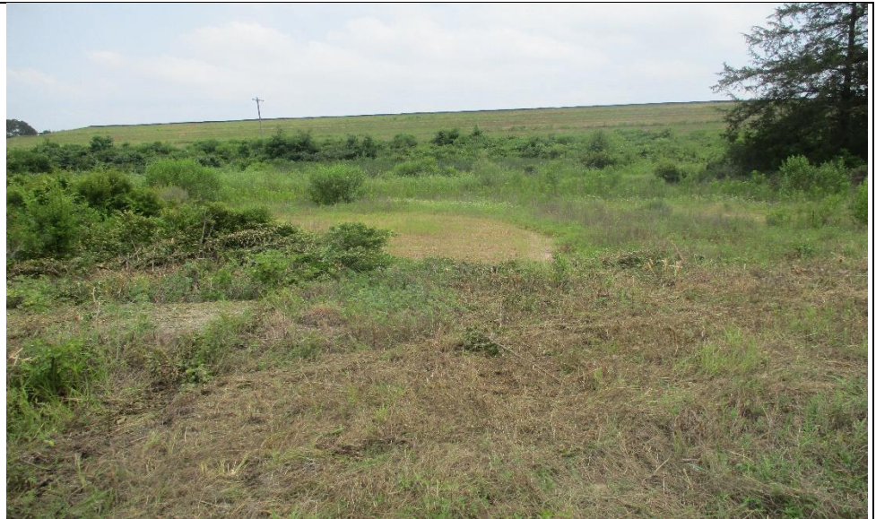
Photograph No. 13 Emergency spillway (looking south)
