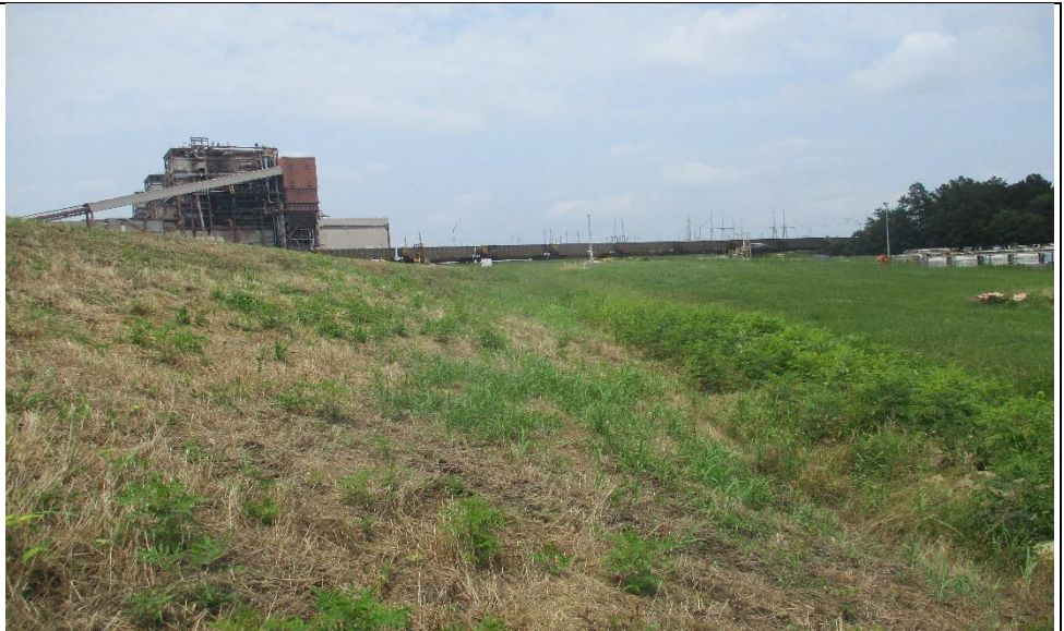
Photograph No. 4 Typical downstream slope (looking north).
