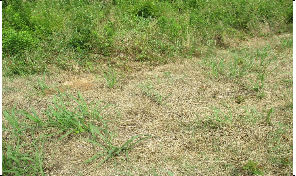
Photograph No. 6 Lower riprap section of the downstream slope.
