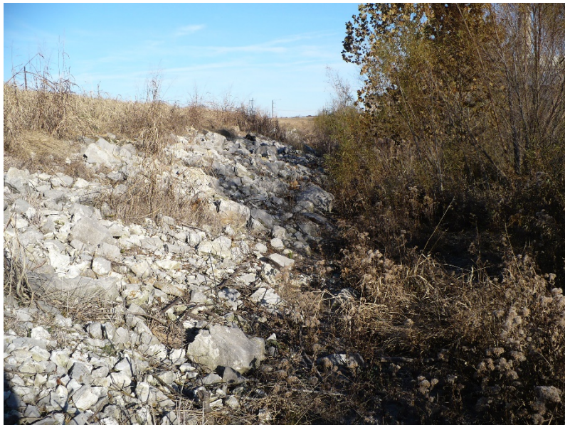
Photo #3 –upstream slope looking towards right abutment
