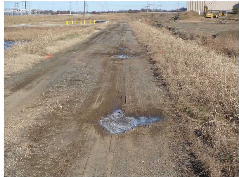
Photo #6 – crest of dam
