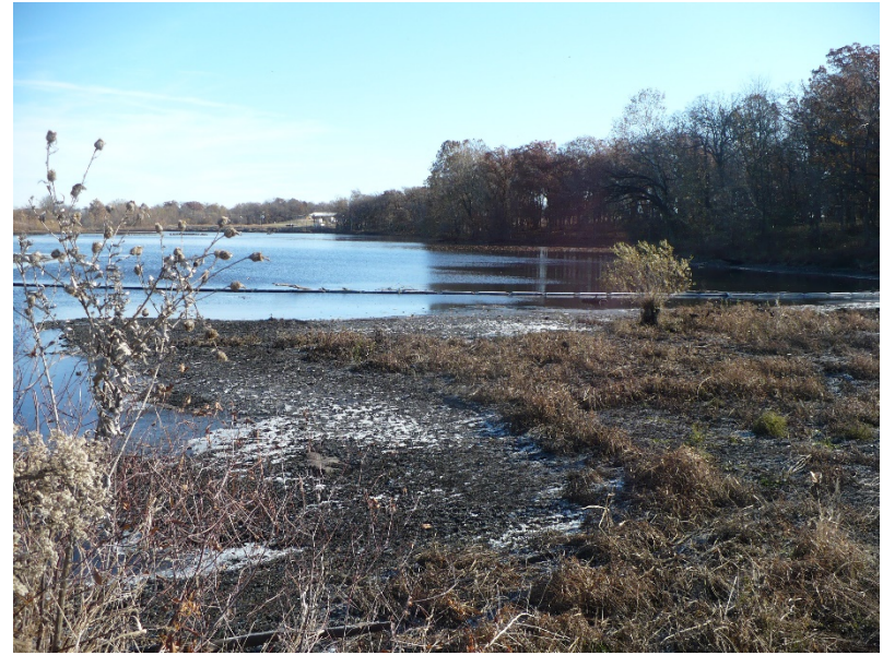
Photo #2 – approach area to emergency spillway
