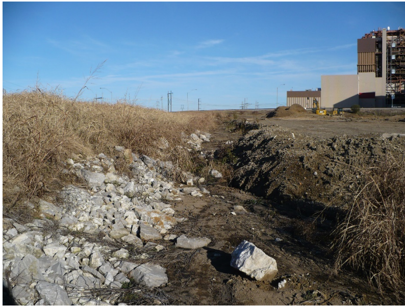
Photo #5 – upstream slope with ash delta
