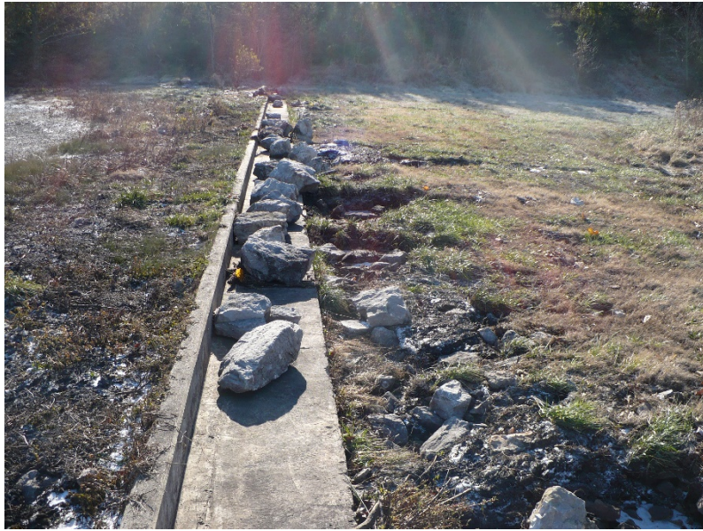
Photo #1 – emergency spillway concrete sill
