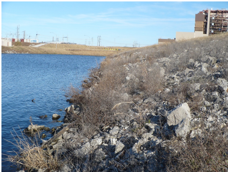
Photo #7 – downstream slope looking towards right abutment
