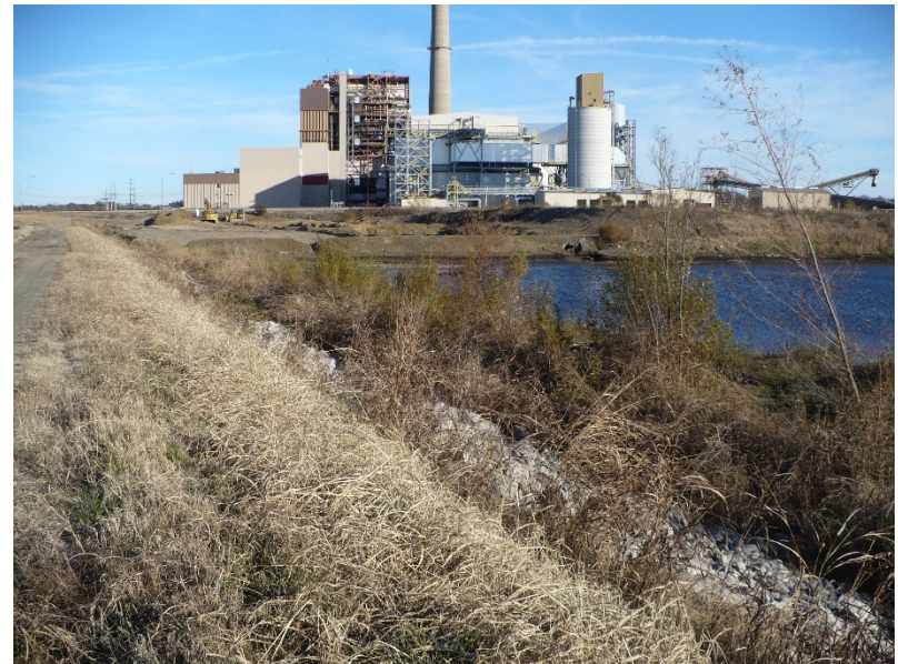
Photo #4 – upstream slope looking towards right abutment
