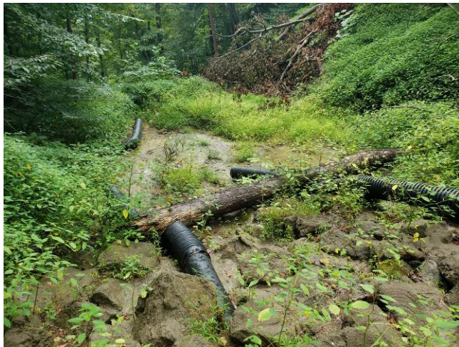
Photograph 11: View of the downstream toe area, showing the outlet of the underdrain pipes.
