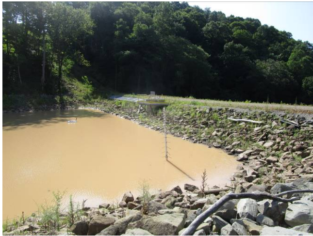
Photograph 10: View of the upstream slope of the south pond dam.
