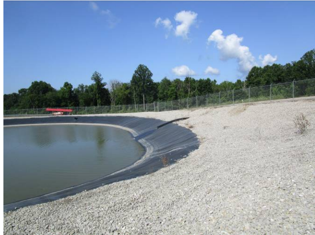
Photograph 13: View of the leachate collection pond.
