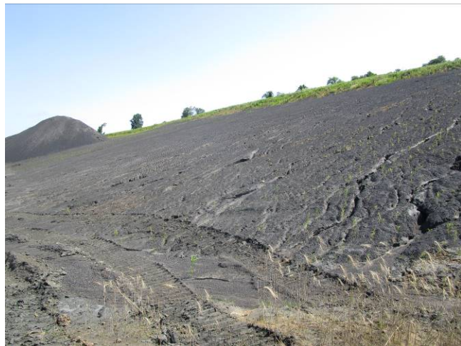
Photograph 2: View of the erosion rills on the protective cover material on the north and east face of the Phase 2 area.
