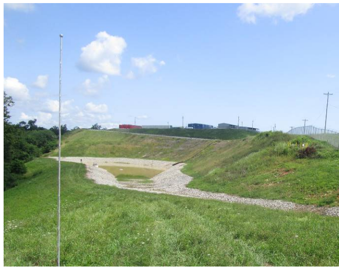
Photograph 14: View of the west pond dam.
