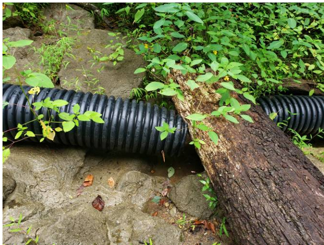
Photograph 12: View of the downstream toe area, showing the outlet of the underdrain pipes.
