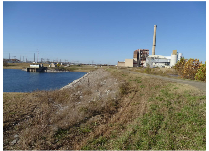
Photo #6 - Downstream slope looking north
