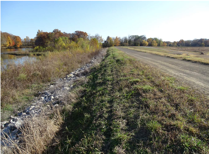
Photo #3 - Upstream slope looking south
