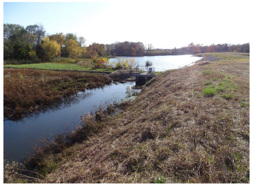
Photo #2 - Principal spillway and approach area to spillway
