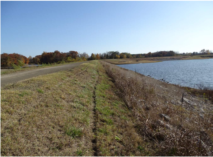
Photo #5 - Downstream slope looking south
