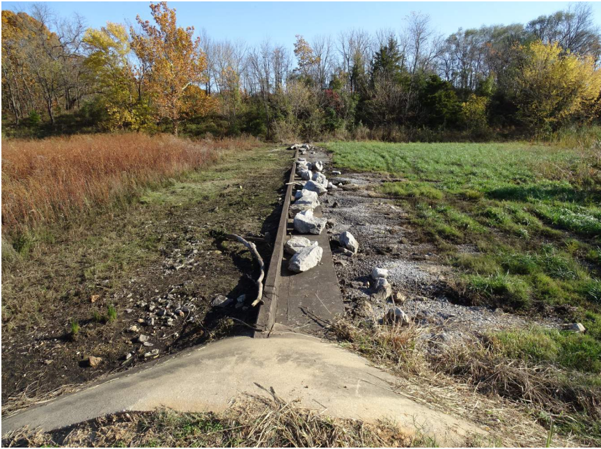
Photo #1 - Emergency spillway concrete sill
