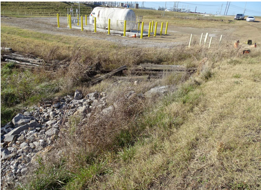
Photo #7 - Right, downstream groin
