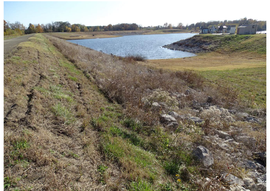
Photo #4 - Downstream slope looking south
