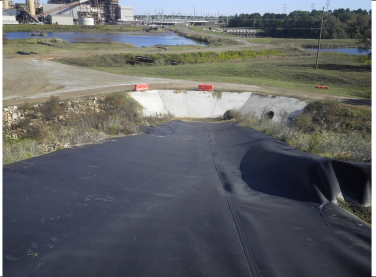
PHOTO #7 HDPE-lined letdown in northeast corner
