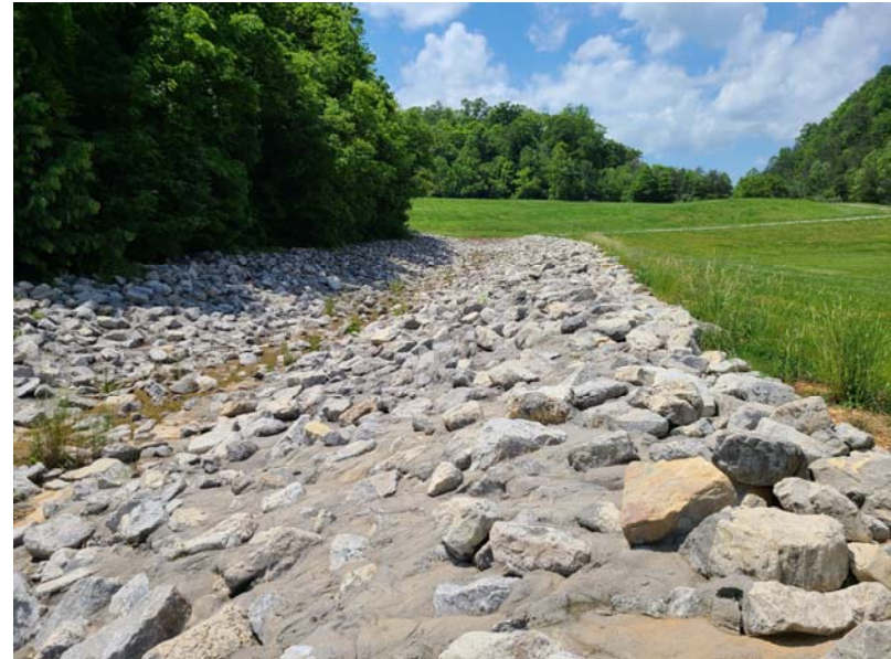
Photo #6 – Pond 1A diversion ditch
