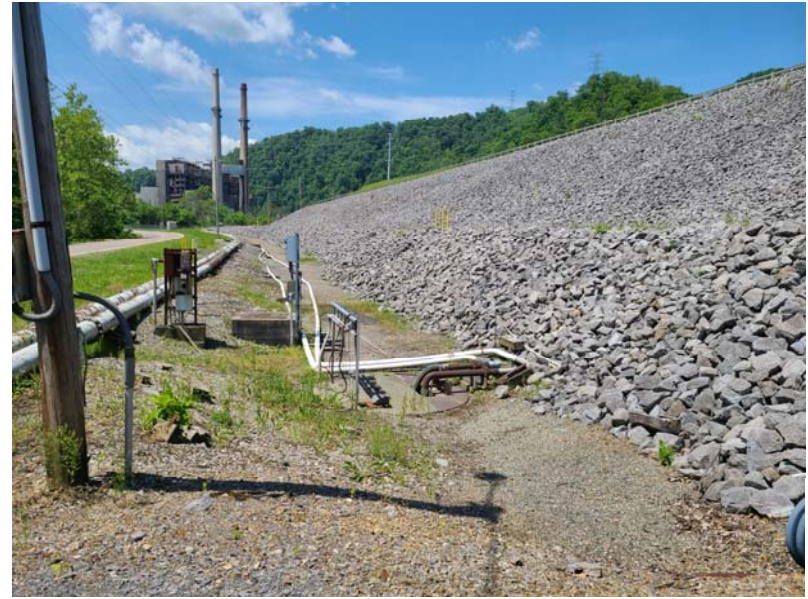
Photo #2 – exterior slopes near transition of 1A and 1B
