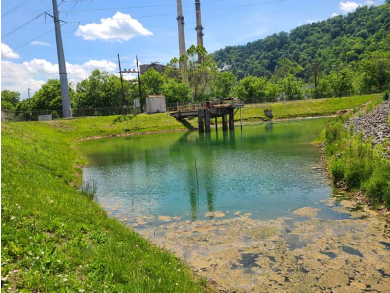
Photo #17 – reclaim pond interior slopes
