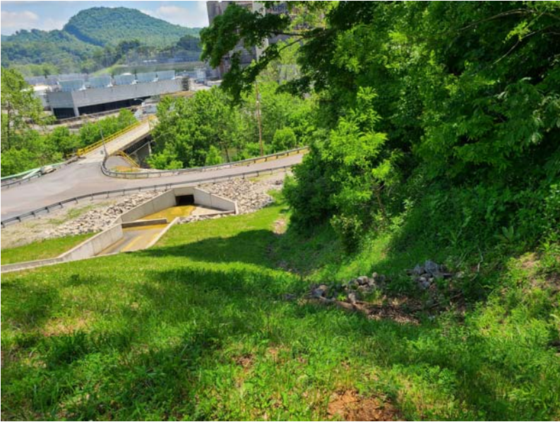
Photo #9 – right abutment, 25-ft clear zone
