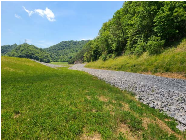
Photo #15 – Pond 1B diversion ditch
