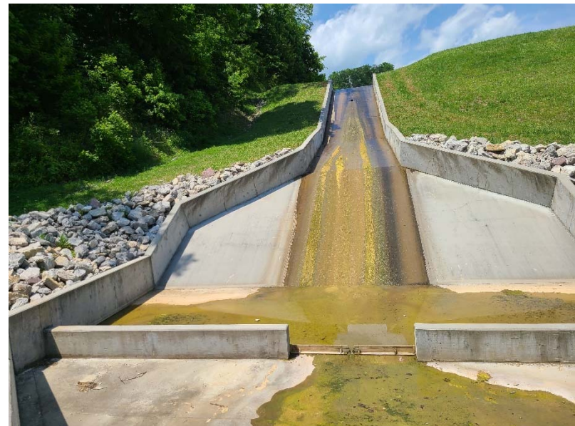
Photo #8 – concrete chute for Pond 1A diversion ditch
