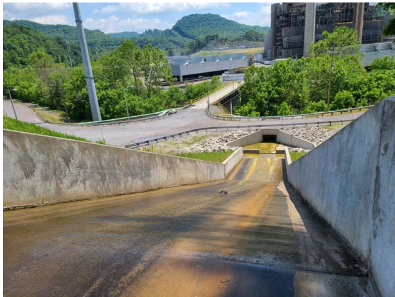
Photo #7 – concrete chute for Pond 1A diversion ditch
