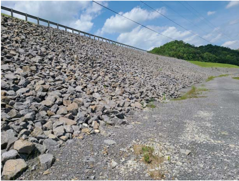
Photo #1 – exterior slopes of Ponds 1A and 1B
