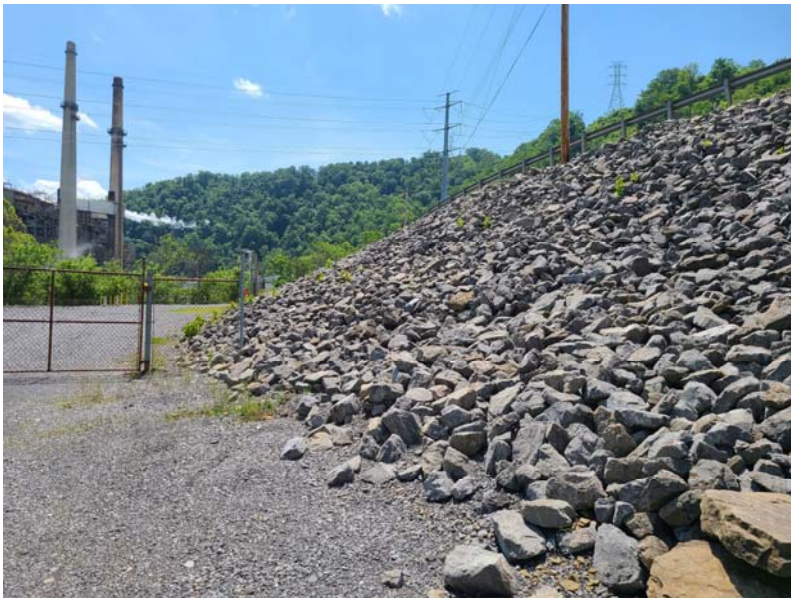
Photo #3 – exterior slope of Pond 1A
