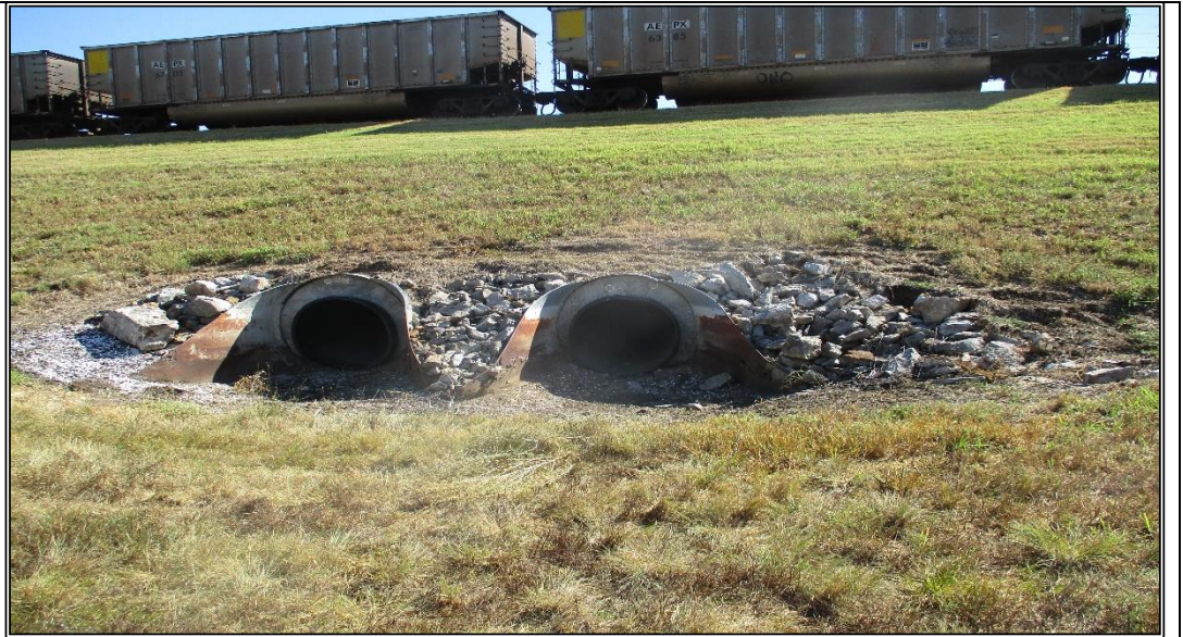
Photograph No. 19 Pipe culverts under the railroad outlet end.
