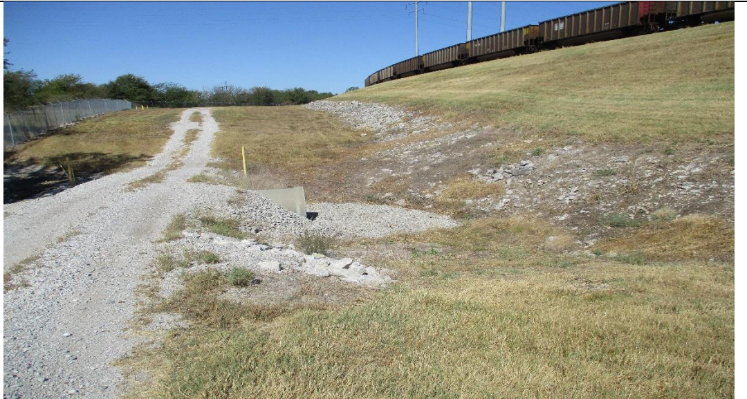
Photograph No. 16 Drainage collection pipe culvert.
