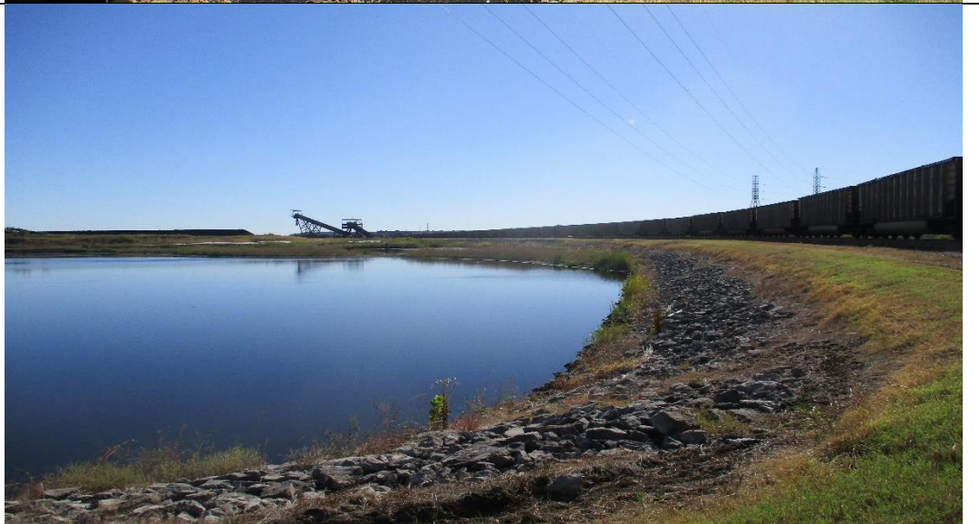
Photograph No. 18 Upstream slope (looking south).
