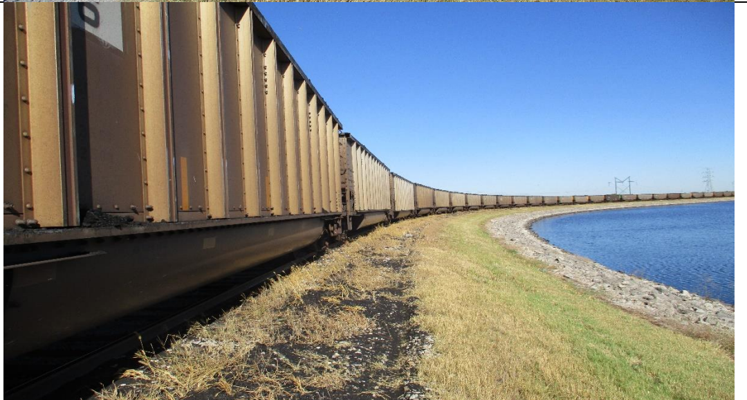
Photograph No. 17 Upstream slope (looking north).
