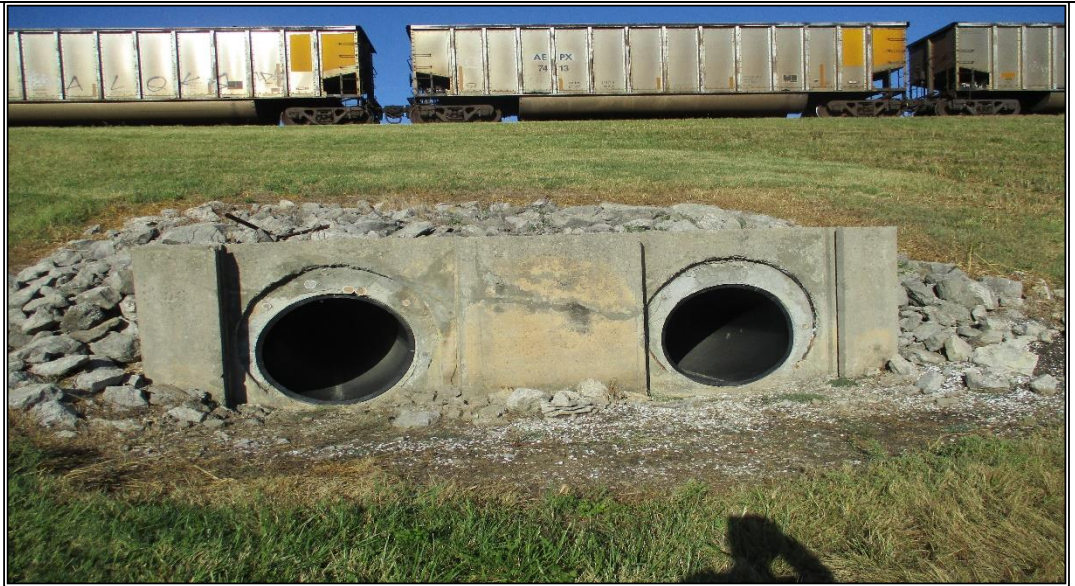
Photograph No. 4 Drainage pipe culverts under the railroad.
