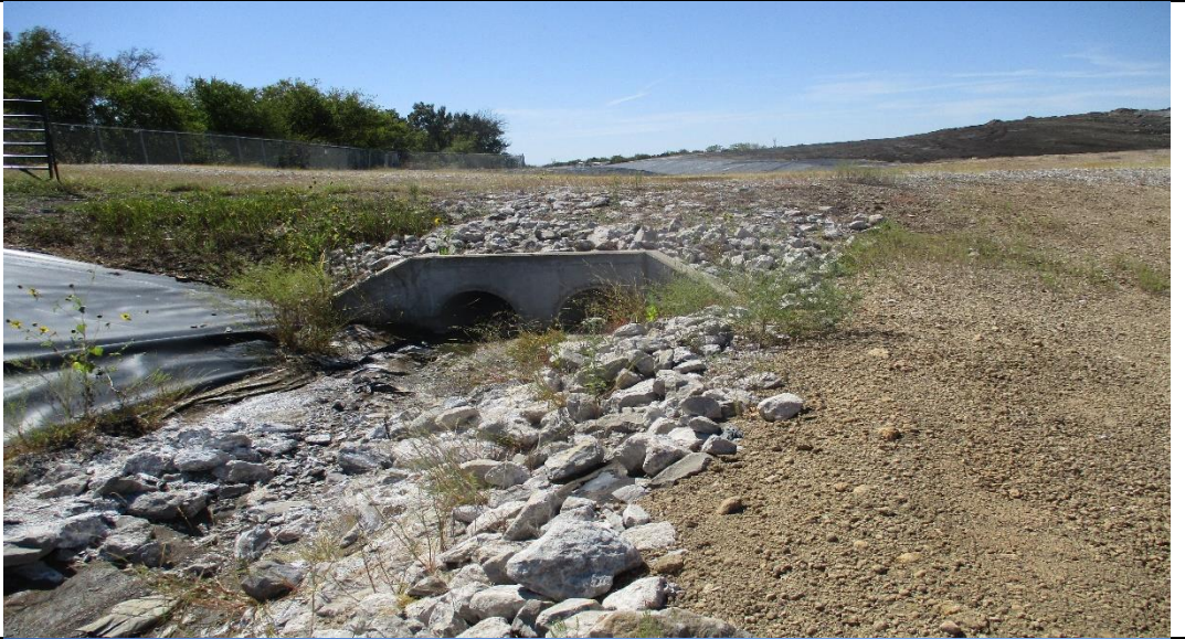
Photograph No. 16 South side perimeter runoff ditch pipe culvert outlet.
