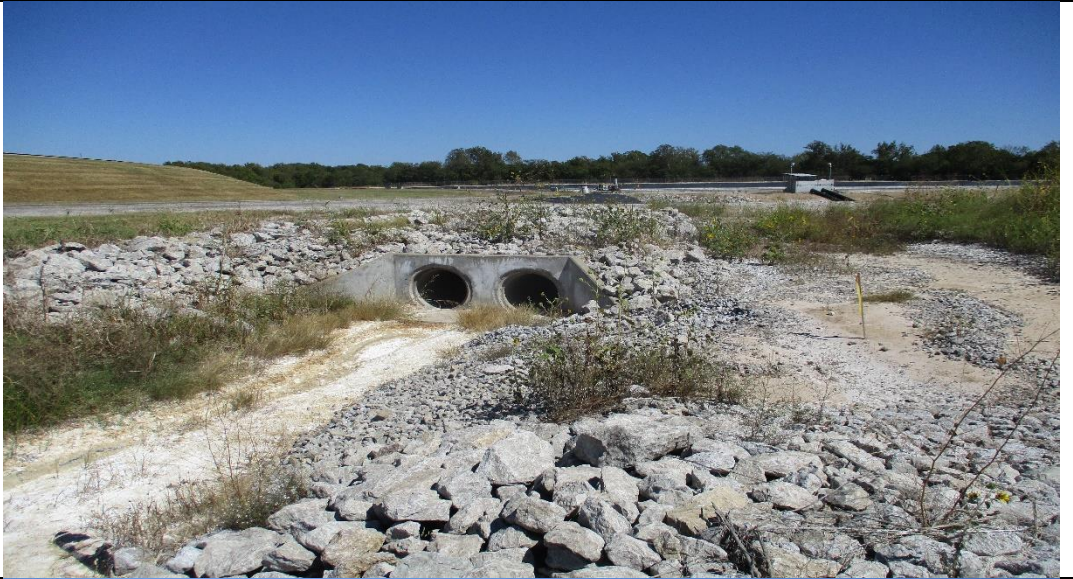
Photograph No. 13 North side perimeter runoff ditch pipe culvert inlet.
