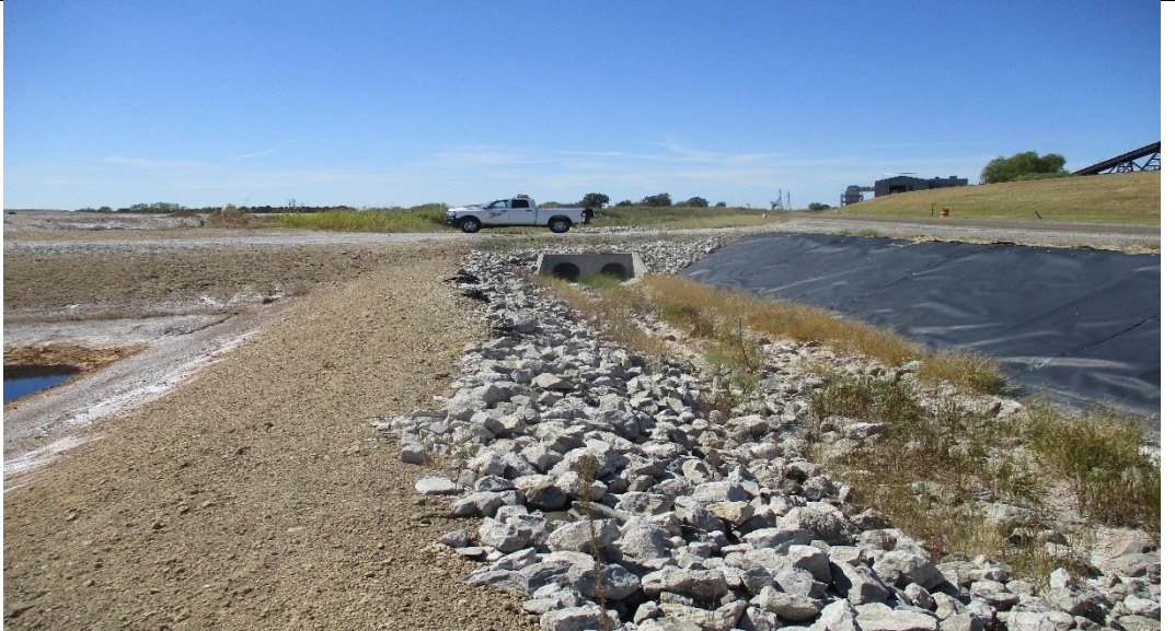
Photograph No. 14 North side perimeter runoff ditch pipe culvert outlet.
