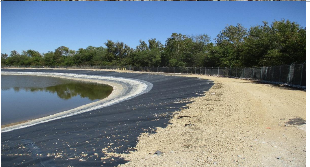
Photograph No. 24 Typical Interior Slope and crest of Basin C.
