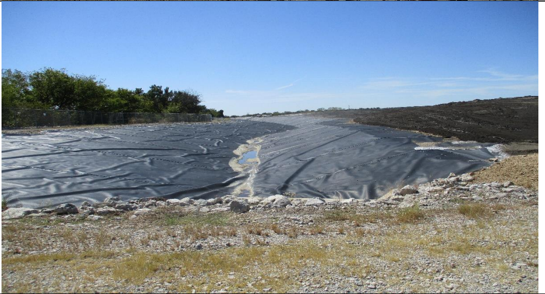
Photograph No. 15 South side perimeter runoff ditch.
