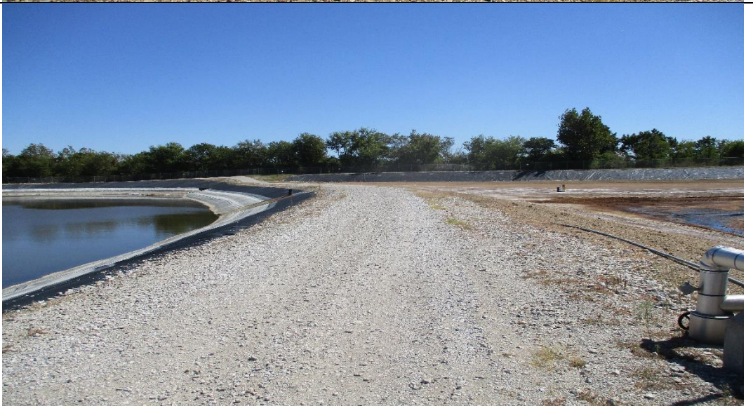
Photograph No. 18 Splitter dike between the leachate pond and Basin C.
