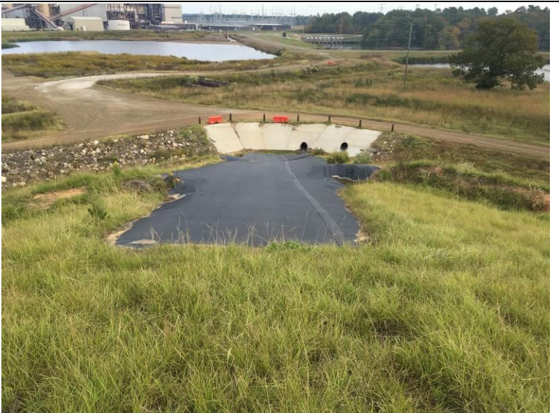
Photo # 7 View of the Northeast Corner Berm Let Down Ditch.
