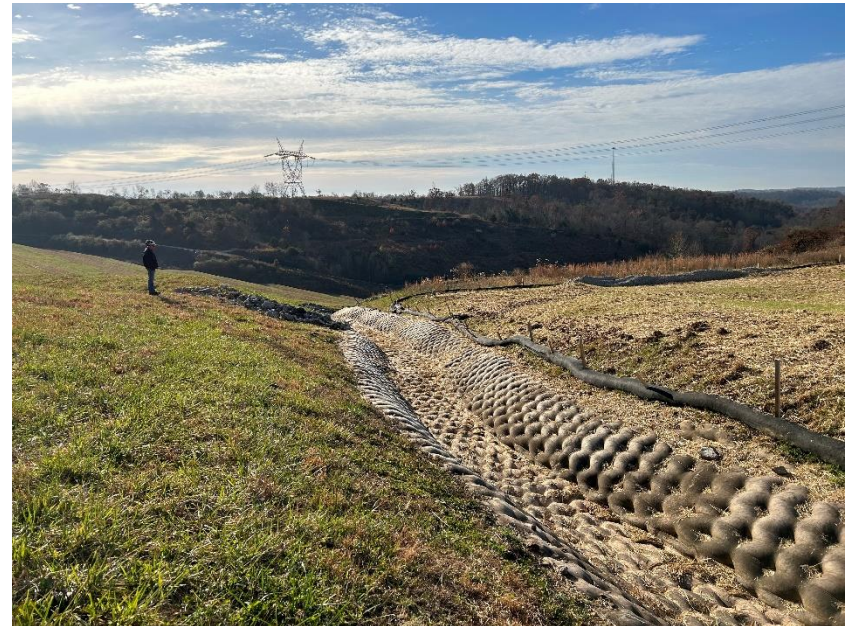
Photo #12 – South Valley Perimeter Ditch-Right Abutment
