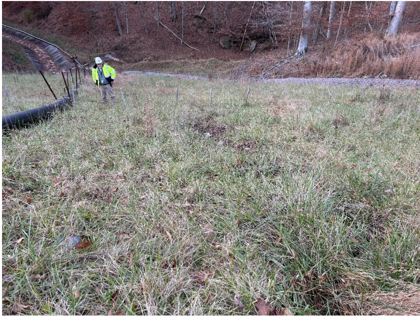
Photo #5 –Sequence 4 North Valley Embankment Slope
