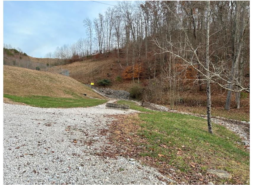
Photo #18 – Outlet Channel from North Valley
