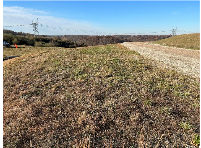
Photo #10 – Covered South Slope-Looking West
