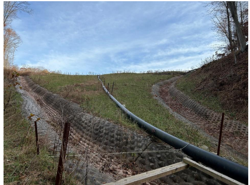
Photo #4 – Photo #4 –Sequence 4 North Valley Embankment Slope
