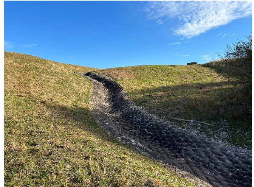
Photo #14 – South Valley Perimeter Ditch-Left Abutment
