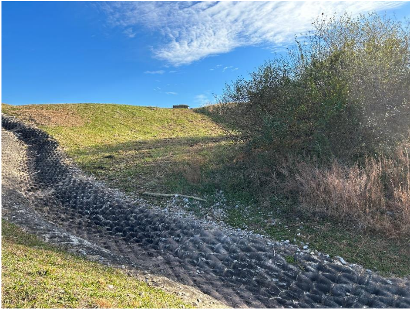
Photo #13 –South Valley Perimeter Ditch-Left Abutment
