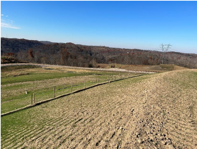
Photo #15 – New Cap/Cover Along 950 Bench
