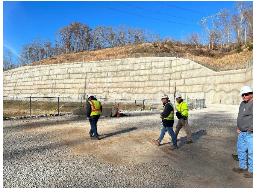
Photo #20 – Soil Nail Wall and Sediment Pond –North Valley
