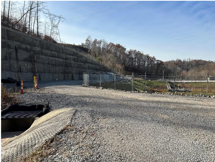
Photo #19 – Soil Nail Wall and Sediment Pond –North Valley
