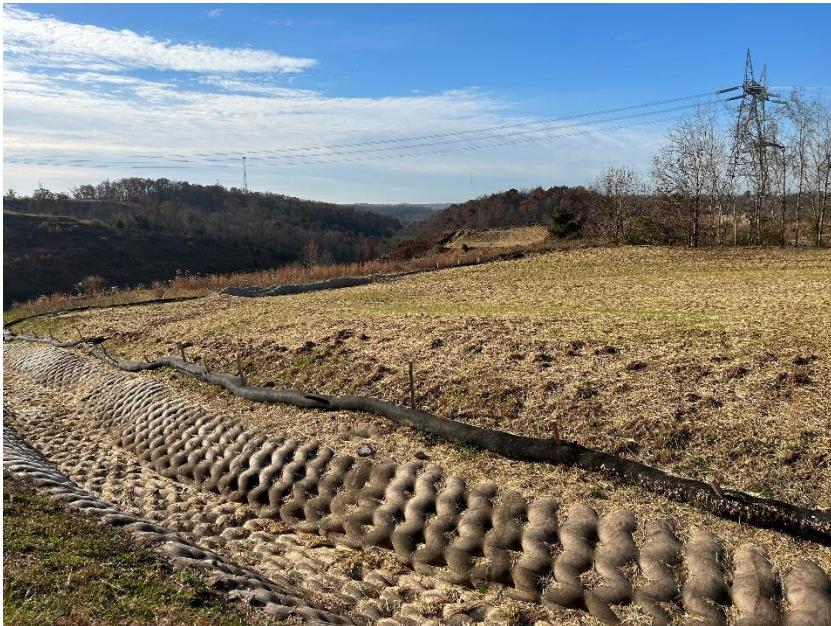
Photo #11 – South Valley Perimeter Ditch-Right Abutment
