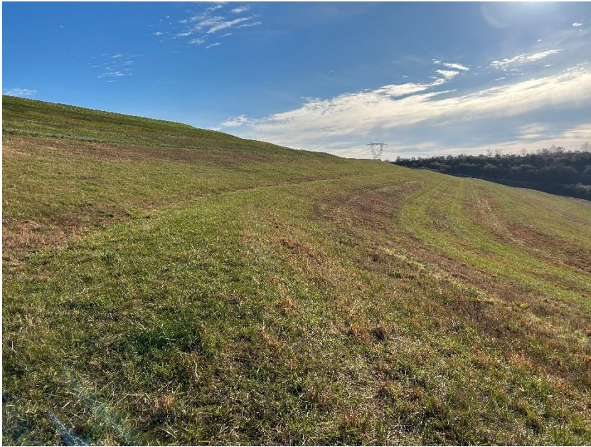
Photo #9 – Covered South Slope-Looking West
