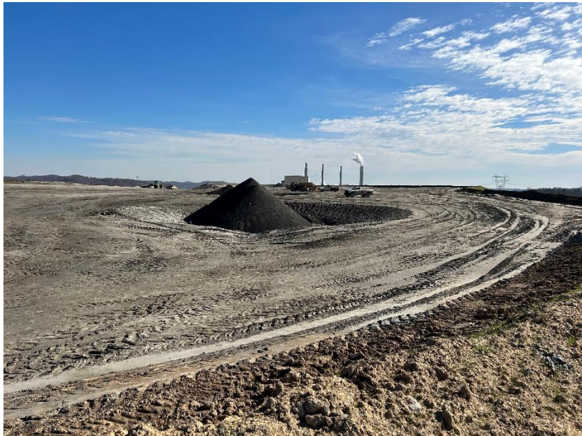
Photo #1 – Chimney Drain in Active Area
