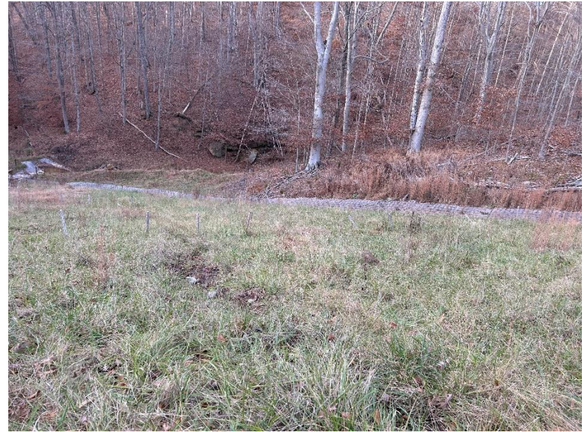
Photo #6 – Sequence 4 North Valley Embankment Slope
