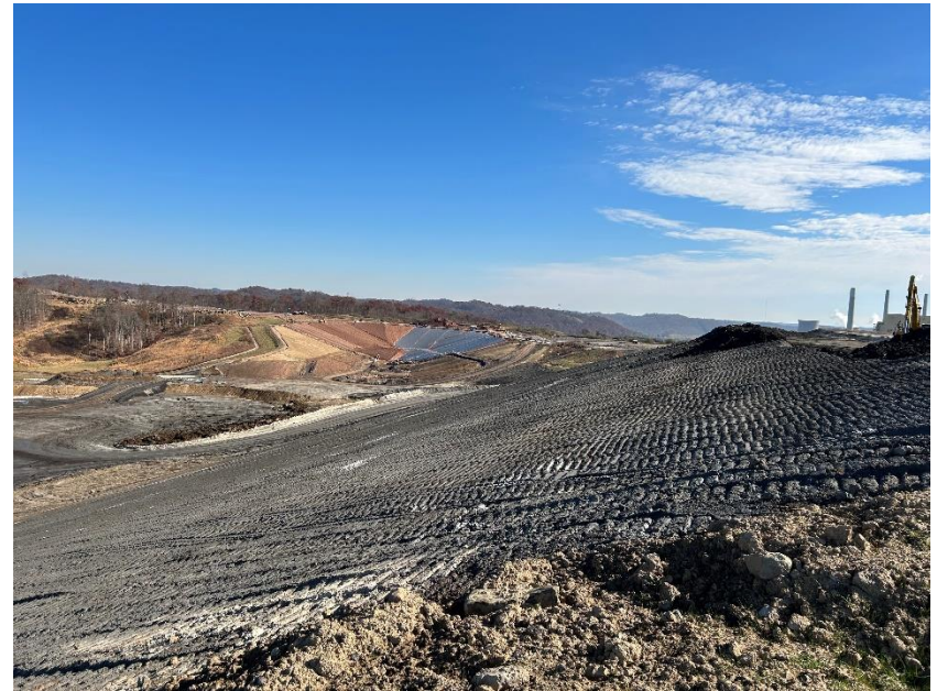
Photo #2 – Crest and Slope in Active Area
