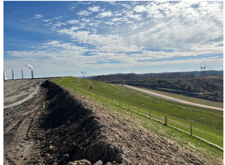
Photo #16 – New Cap/Cover Along 950 Bench
