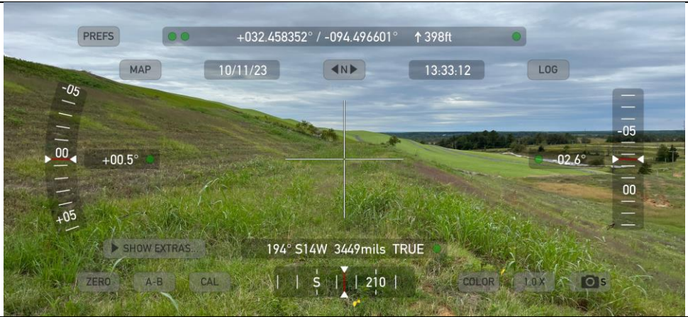
Photograph No. 30 View of cell 2005 showing vegetative final cover. (looking southwest)
