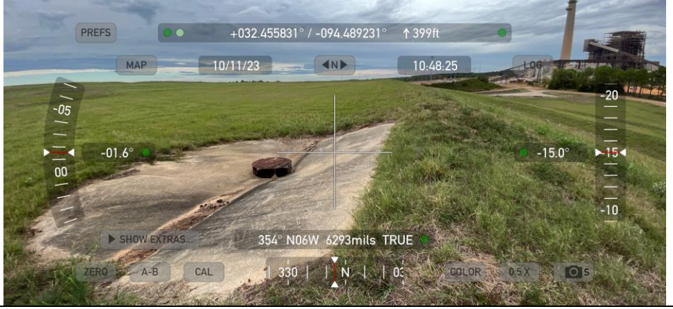
Photograph No. 3 Typical condition of the vegetative cover over the northwestern areas of the landfill cap. View of the Cell 1984 let-down catch basin (looking northwest)
