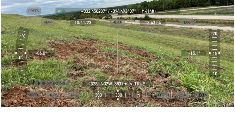
Photograph No. 33 Damage from hog activity was observed at exterior slope of Cell 1995. (looking northwest)
