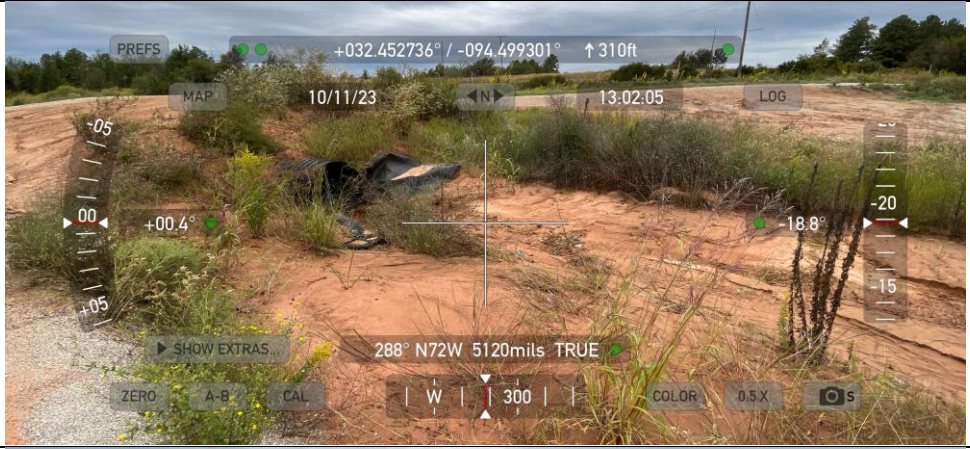
Photograph No. 27 Vegetation and sedimentation build up was observed at western side of let down ditch near cell 2015.
