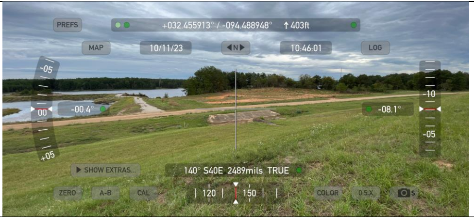
Photograph No. 1 View of the storm water let-down pipe on the east side of the landfill area. (looking southeast)
