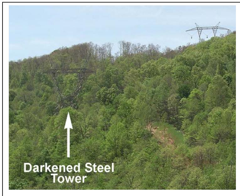
Figure 8. Darkened Steel Transmission Towers Before Wire is Installed
