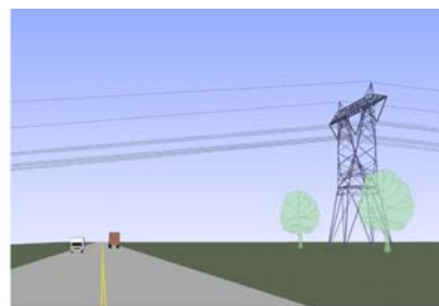
765 kV One Single Circuit Tower (200 ft. Right-of-Way)
