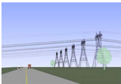
345 kV Six Single Circuit Towers (900 ft. Right-of-Way)
