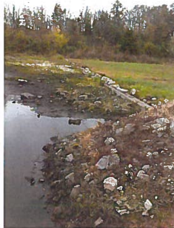
Photo 2 – emergency spillway concrete weir
