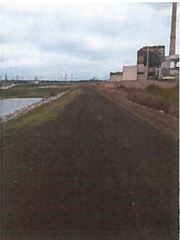
Photo 5 – crest – looking towards right abutment
