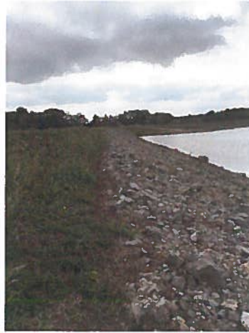
Photo 8 – downstream slope – riprap and grassed surface
