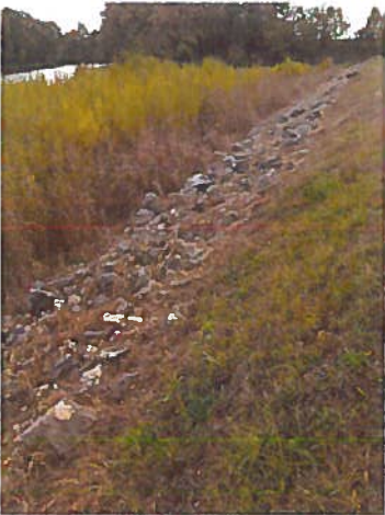
Photo 3 – upstream slope – riprap and grassed surface.
