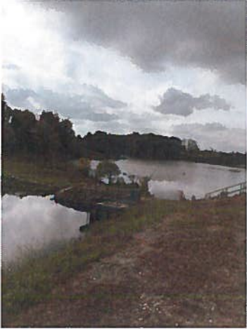
Photo 1 – principal spillway structure
