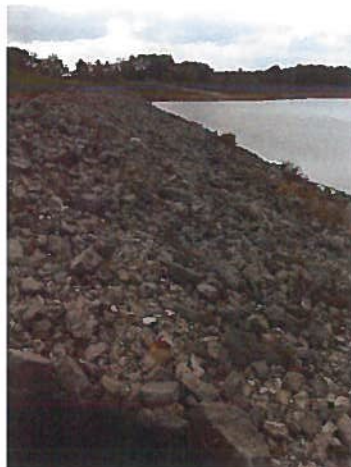
Photo 6 – downstream slope – looking towards left abutment
